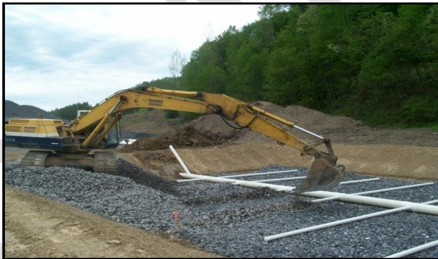
Figure 7.9. Limestone being placed on top of the underdrain piping system
