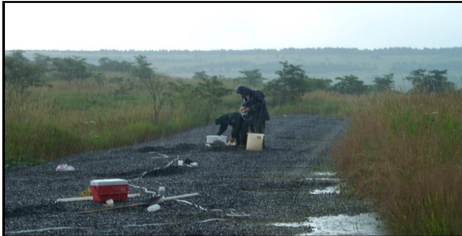
Figure 7.3. Typical Manganese Removal Bed
