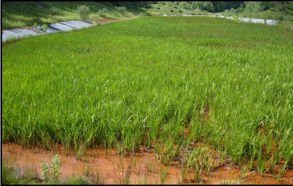
Figure 7.2. Synthetically-lined wetland used in removing low concentrations of suspended iron
