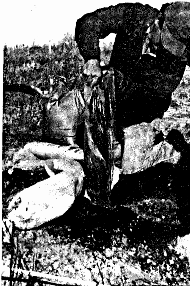
FIG. 5-13: LOADING OF IREGEL SLURRY EXPLOSIVE IN BLASTHOLE
