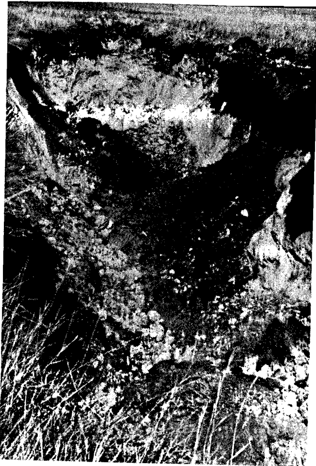
FIG. 10-4: VIEW OF BLAST #1 (N-14) IMMEDIATELY AFTER BLASTING
