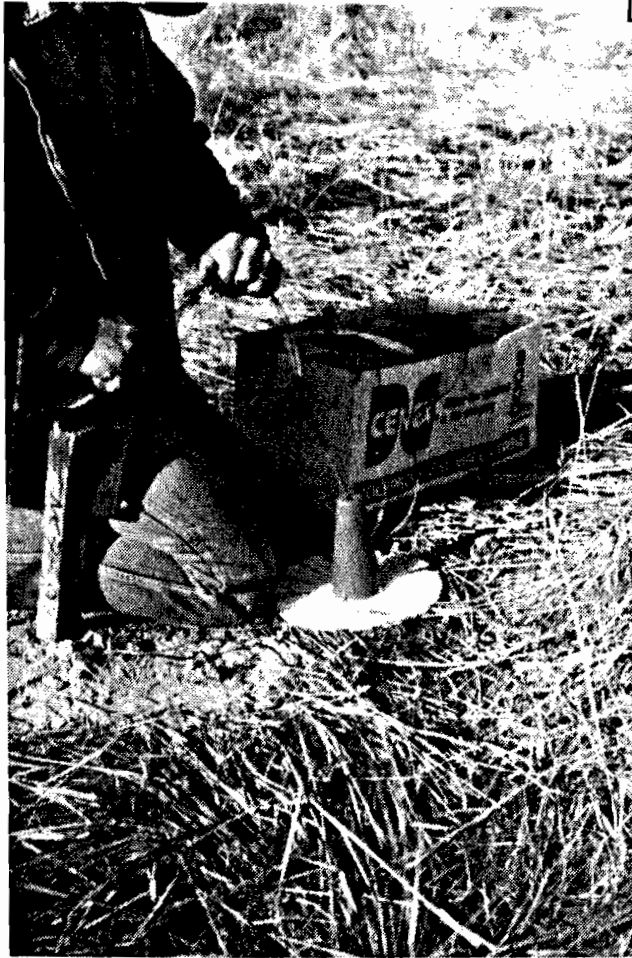
FIG. 5-2: ILLUSTRATING USE OF BALER TWINE TO HOLD PLASTIC HOLE PLUG IN POSITION IN BLASTHOLE
