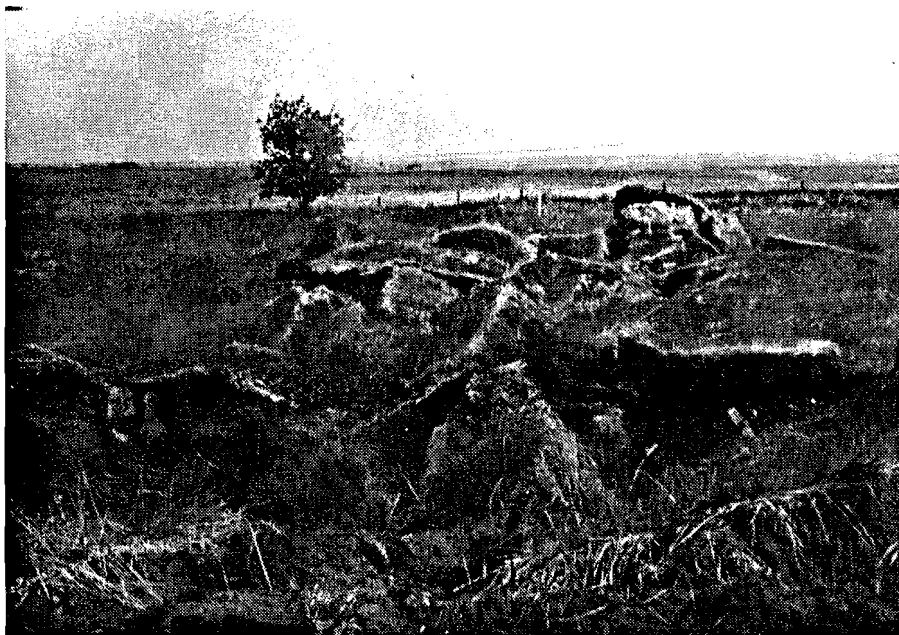
FIG. 4-21: POST-BLAST PROFILE OF BLAST #18 (N-6), LOOKING NORTH
