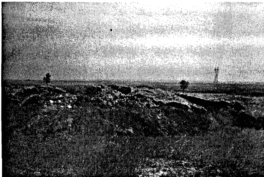
FIGURE 4-11: POST-BLAST PROFILE OF BLAST #4(N-1, N-2) LOOKING NORTH
