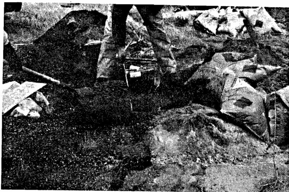
FIG. 5-11: BACKFILLING A BLASTHOLE TO POSITION OF LOWERMOST EXPLOSIVE DECK USING CRUSHED ROCK STEMMING MATERIAL
