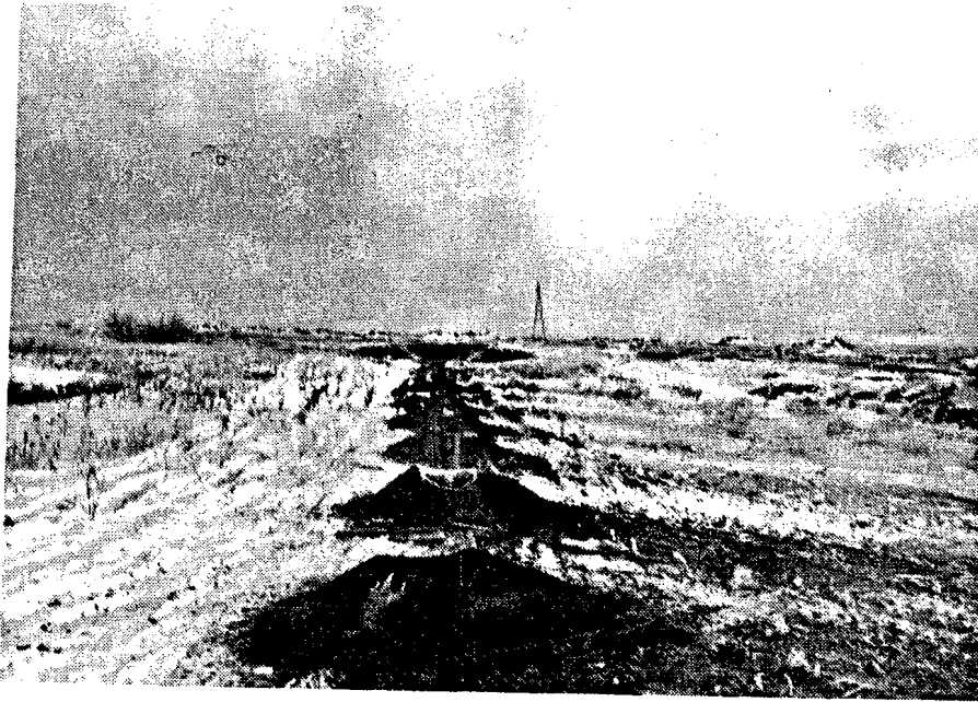
FIG. 4-24: PRE-BLAST VIEW OF BLAST #21 (S-9(S)), LOOKING NORTH, PRIOR TO LOADING
