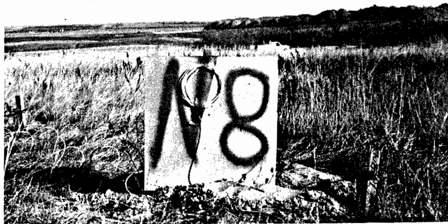
FIG. 6-2: ILLUSTRATING COMMON PRACTICE FOR HIGH-SPEED CAMERA TARGETS - SINGLE COIL OF NONEL TRUNKLINE ATTACHED TO ONE DECK IN A BLASTHOLE
