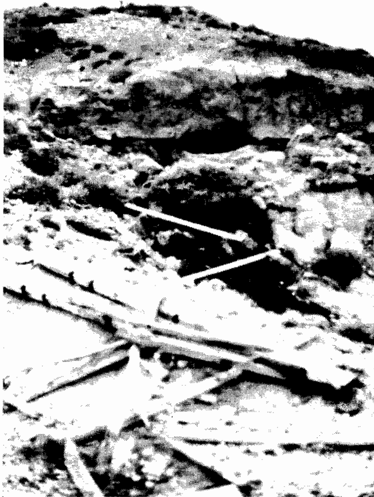
FIGURE 5-7: ADIT PROVIDING ENTRY TO THE UNDERGROUND WORKINGS SHOWING THE SMALL OPENING NEAR THE TOP OF THE ADIT
