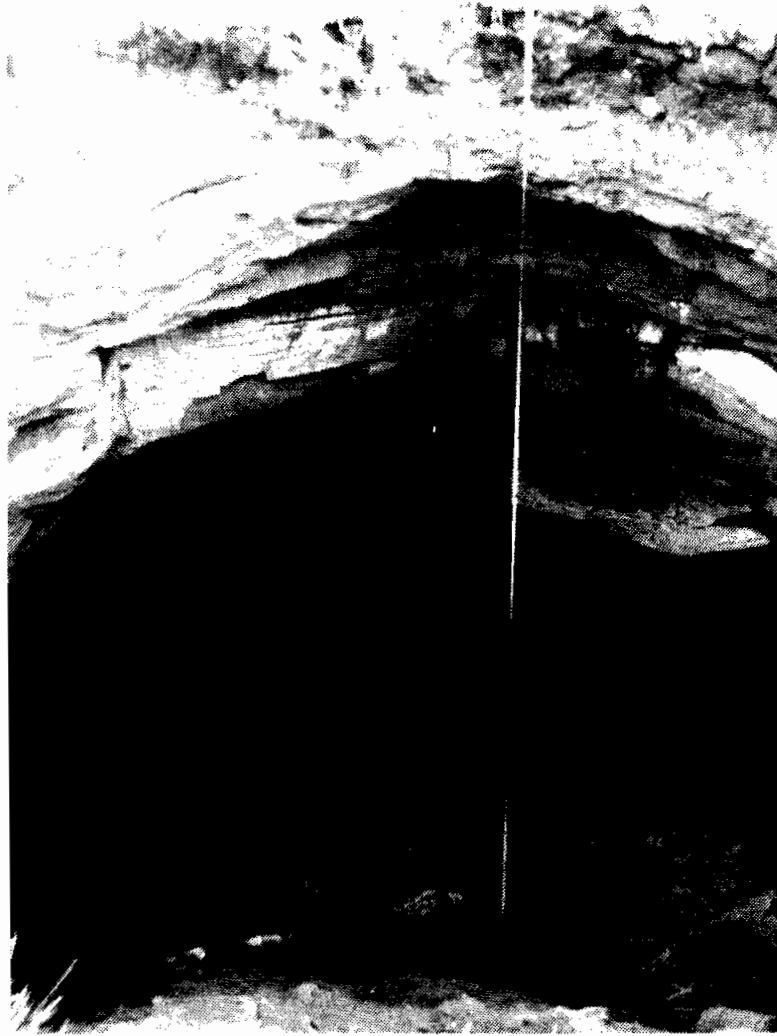
FIGURE 4-23: VIEW OF VO-12 SHOWING THE LARGE, SLOPING VOID STRIKING EAST
