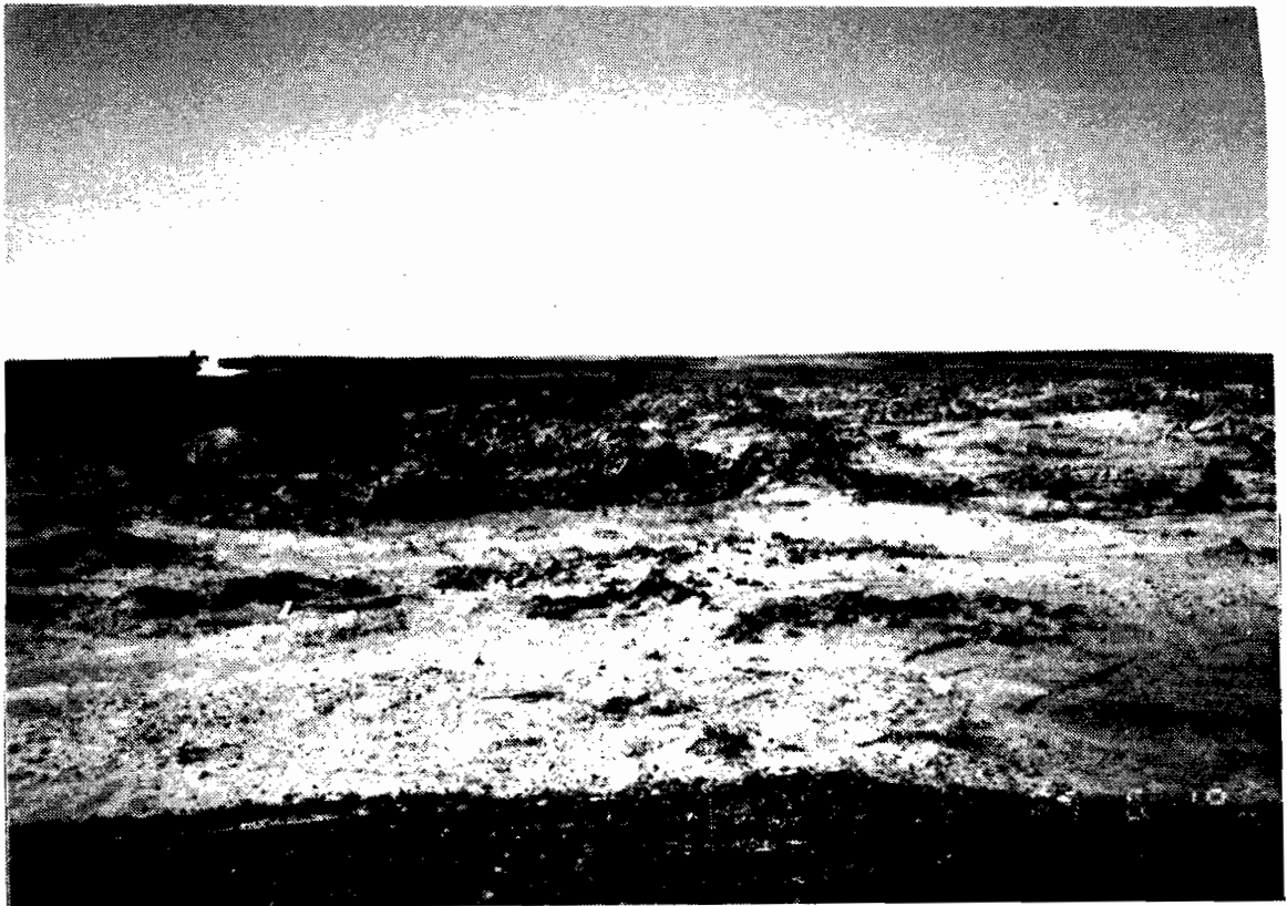
FIGURE 5-13: VIEW OF B7 AFTER BLASTING LOOKING SOUTH WITH B7 IN THE FOREGROUND
