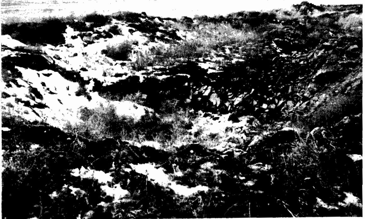
FIGURE 4-15: FINAL RESULT AT THE SOUTH END OF VO-7 AFTER TWO BLASTS
