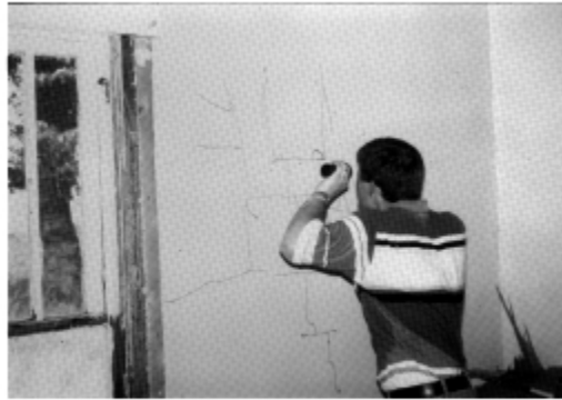
Figure 28. Visual inspections for cracking at the Shack. A 7-power optical magnifier and sidelight are being used. Preexisting cracks before the study were highlighted with marker.
