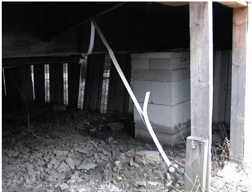
Figure 2 Hurricane straps required by building code in states in which trailer were selected for the study in Ohio, Tennessee, Alabama, and Indiana
