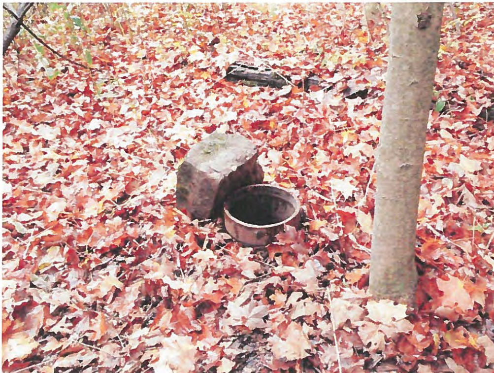
Photo 1. WPC 3 well (note the open, exposed casing - the rock has since been placed on top to cover the opening).
