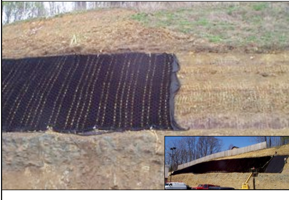
...CCS panel installation continues across slope...
