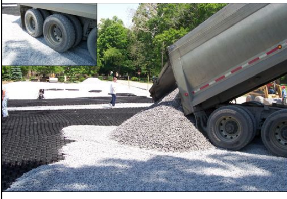
Infill is placed onto expanded CCS.
