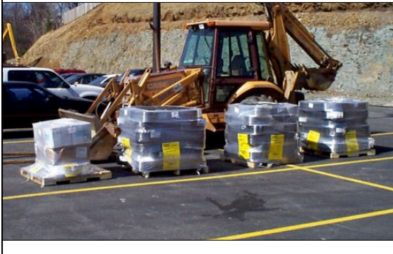
...palletized, unexpanded CCS was delivered to project site...
