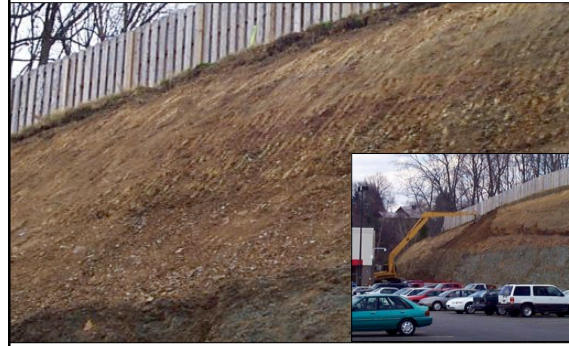
...loose rock and soil was removed to prepare the surface...
