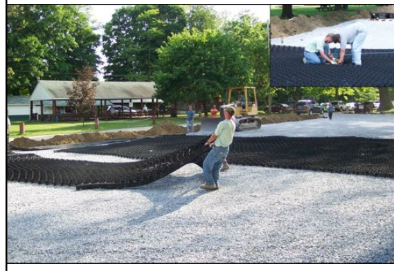
CCS panels are expanded and stapled.
