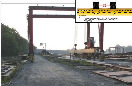
Rutting of unconfined gravel caused costly maintenance problems for both the yard and equipment
