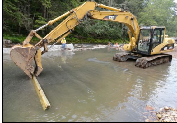
The stone base was leveled prior to ACB mat placement.
