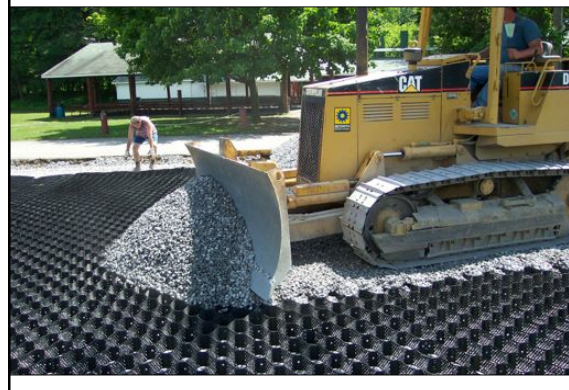
Infill is spread and compacted into CCS.
