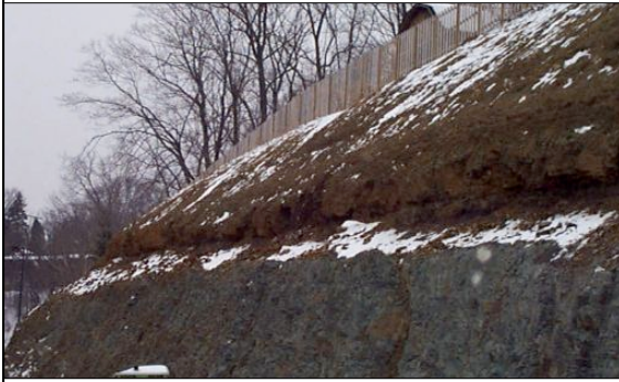
Rocks falling from the slope face onto the parking lot was the problem...
