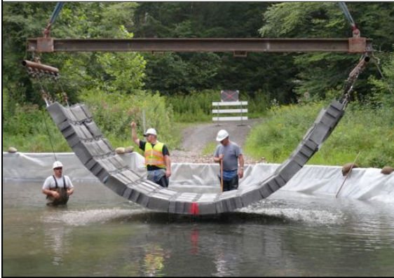
The ACB System installation sequence continues.
