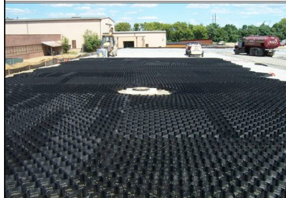
Panels are easily fit around protrusions.
