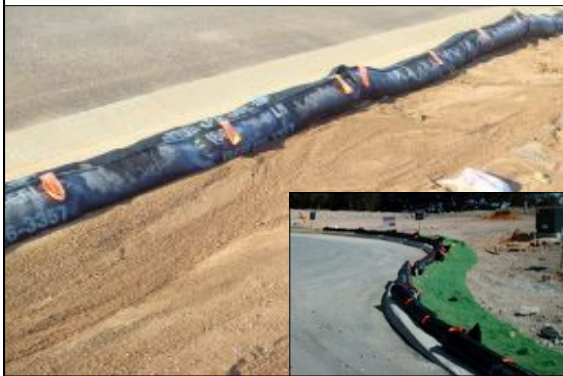
Weighted Sediment Tubes: Perimeter Controls
