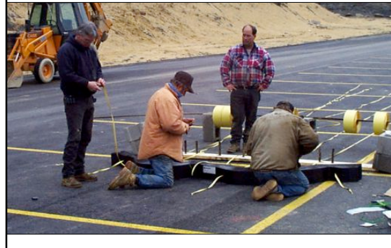
...apparatus was created to run tendons through CCS panels...
