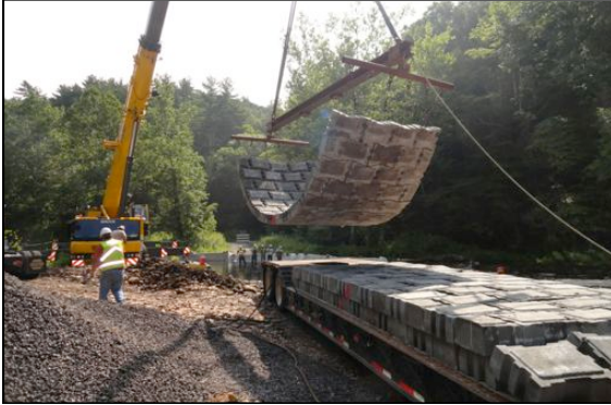
ACB Mat Placement Sequence begins as mats are picked up from the flatbed using a Spreader Bar.
