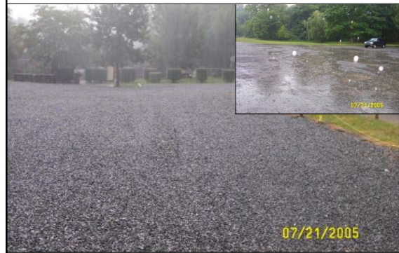
Comparison of CCS gravel parking area vs conventional gravel lot during a rain event.
