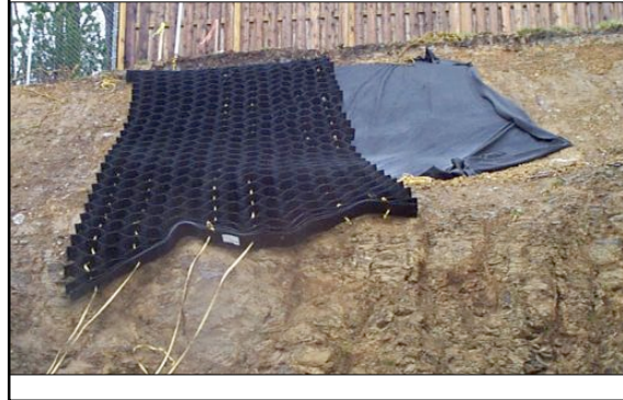
...Geotextile fabric was placed first and then CCS panels with tendons secured to anchor I-Nuts ...
