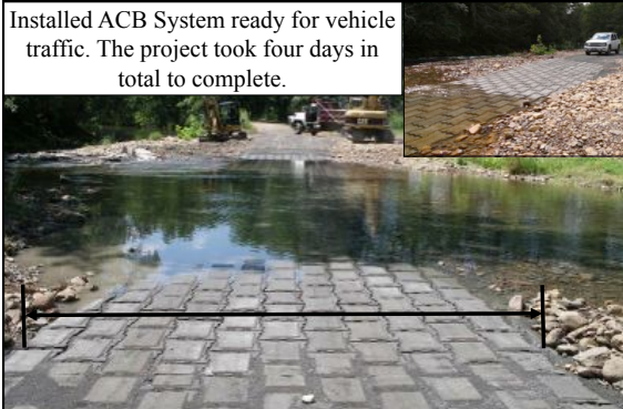
The ACB mats were fabricated to meet the specified 14' travel lane width.
