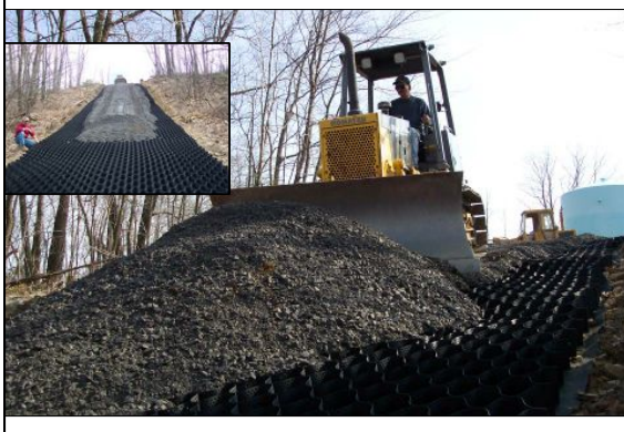
Filling cells with a 2A stone w/ 2" wearing surface
