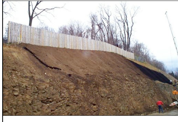
...view of partially in-filled CCS on slope...
