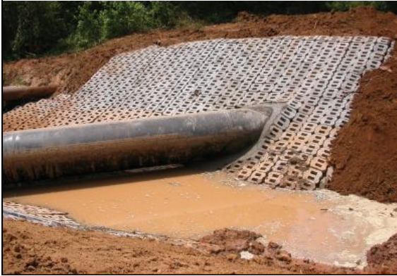
Pipe Protrusions
