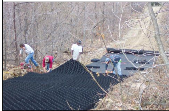
Expand panels and anchor in place.
