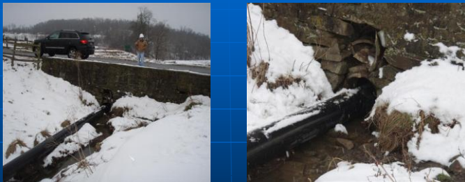
Running utility lines through existing culverts
