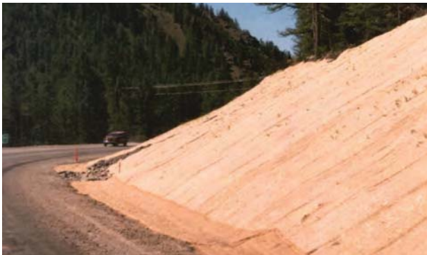
Every site has its own unique characteristics and challenges. EroNet Erosion Control Blankets are available in varying longevities to suit a variety of scenarios and conditions.
