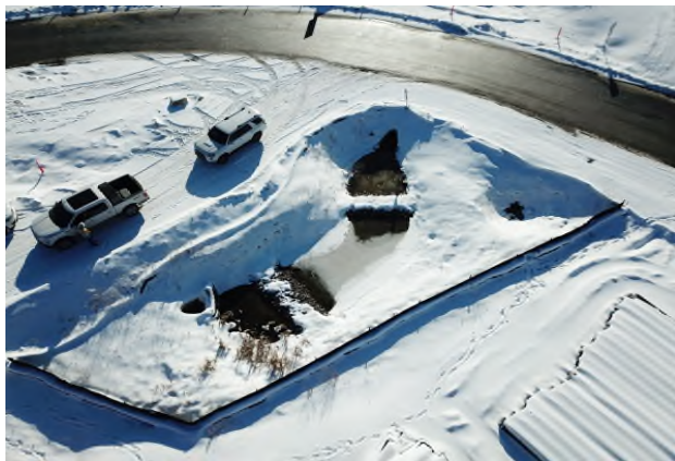
Photo # 35 : 01/28/2019-- Stream O43 and Pond O2 Upstream (aerial)
