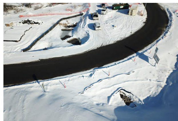
Photo # 36 : 01/28/2019-- Stream O43 and Pond O2 Upstream (aerial)
