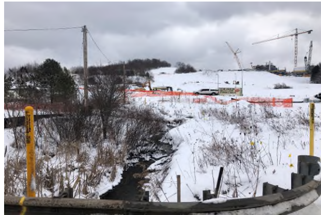
Photo # 28 : 01/27/2019 -- Stream 044 UNT to Hinckston Run (CWF) Facing east or upstream along O44 on the eastern side of William Penn Ave (SR-271). Orange safety fence is unrelated to Mariner East II project.
