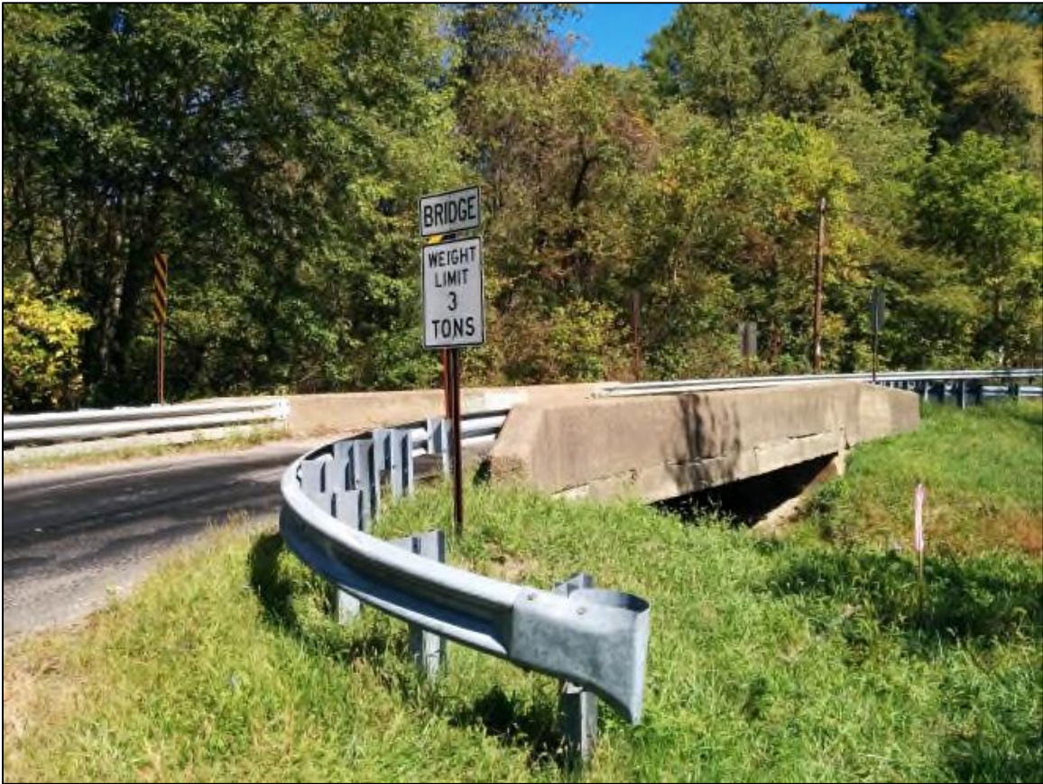
Ullom Road Bridge over Westland Run Facing Northeast
