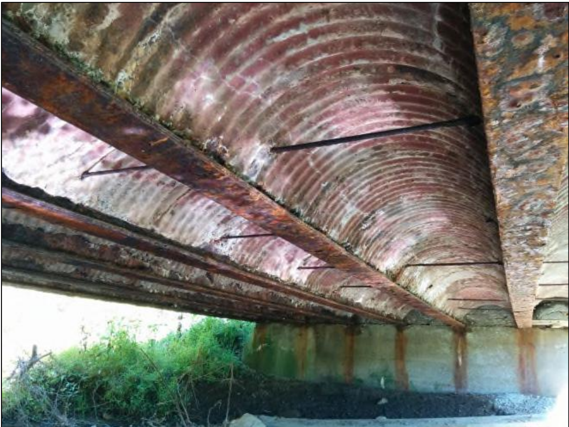
Underside of Ullom Road Bridge
