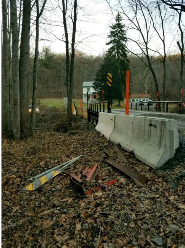
Photo 5 – 12/18/2017 – Looking northwest across bridge.
