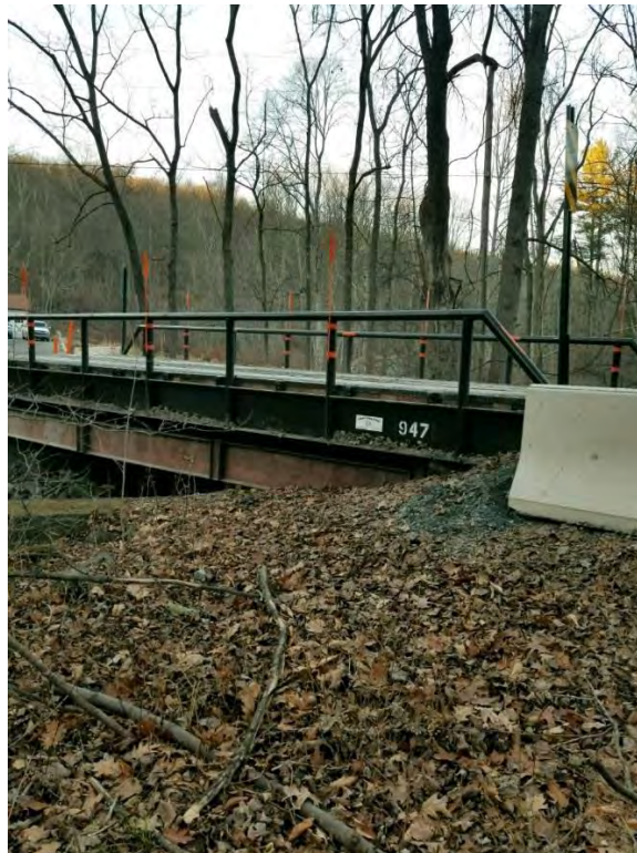
Photo 4 – 12/18/2017 – Looking southeast at bridge.
