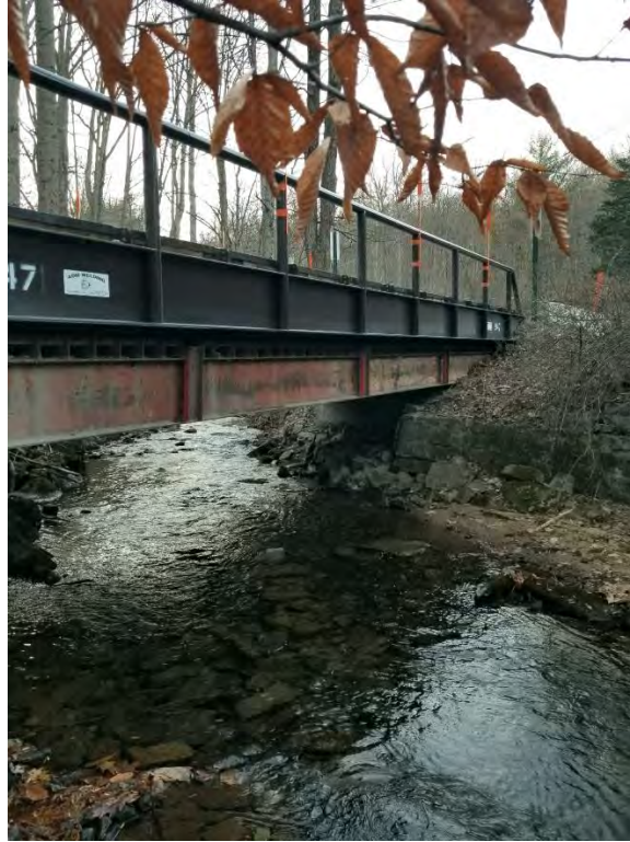
Photo 1 – 12/18/2017 – Looking southwest at bridge.
