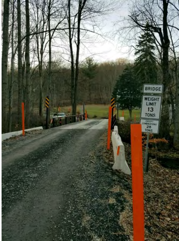
Photo 3 – 12/18/2017 – Looking west across bridge.
