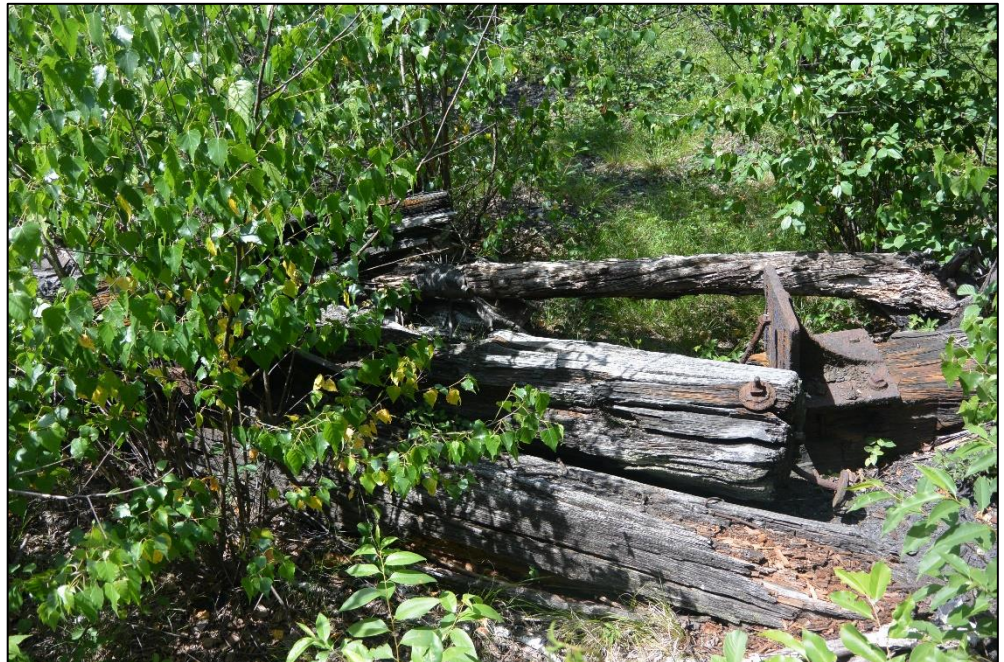
Figure 5: No.14 Shaft, derelict structures 30ft east of mapped shaft location. June 2016
