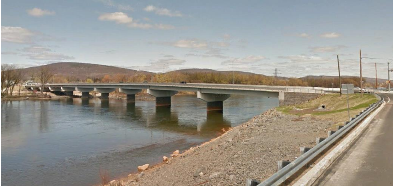
Figure 3-2 The Wyoming Bridge
