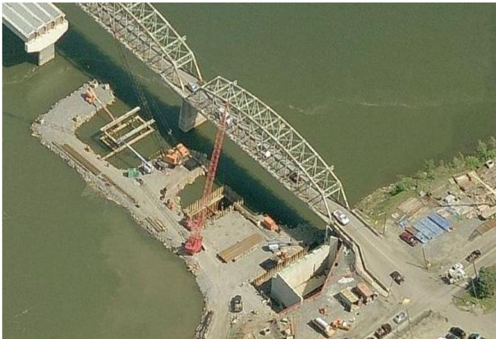
Figure 4-1 Sheet Pile Cofferdams Used to Construct the Wyoming Bridge
