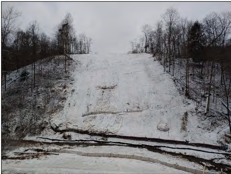
Looking upslope at station 1311+00
