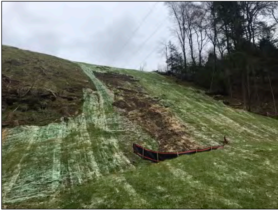
Looking south towards CIS Elkhorn Run Road near station 888+00
