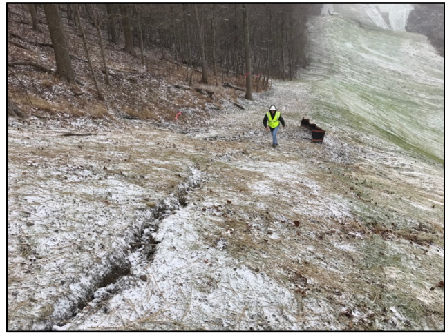
Looking West along Pipeline ROW at Elkhorn Run Site 1.
