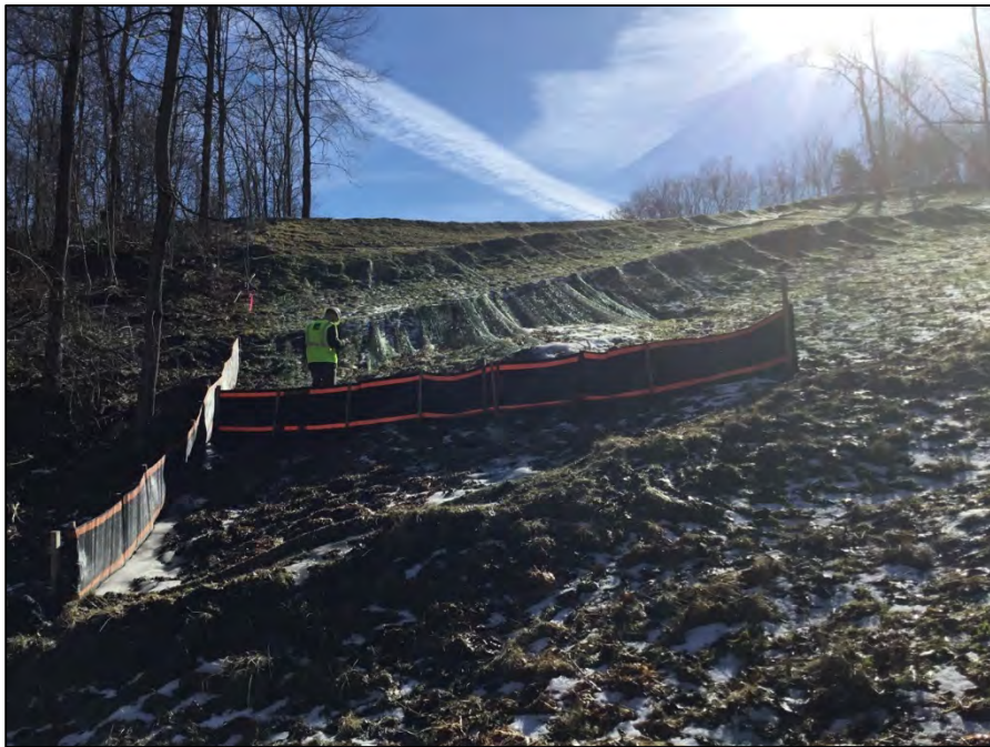
Looking south towards feature near station 1868+50
