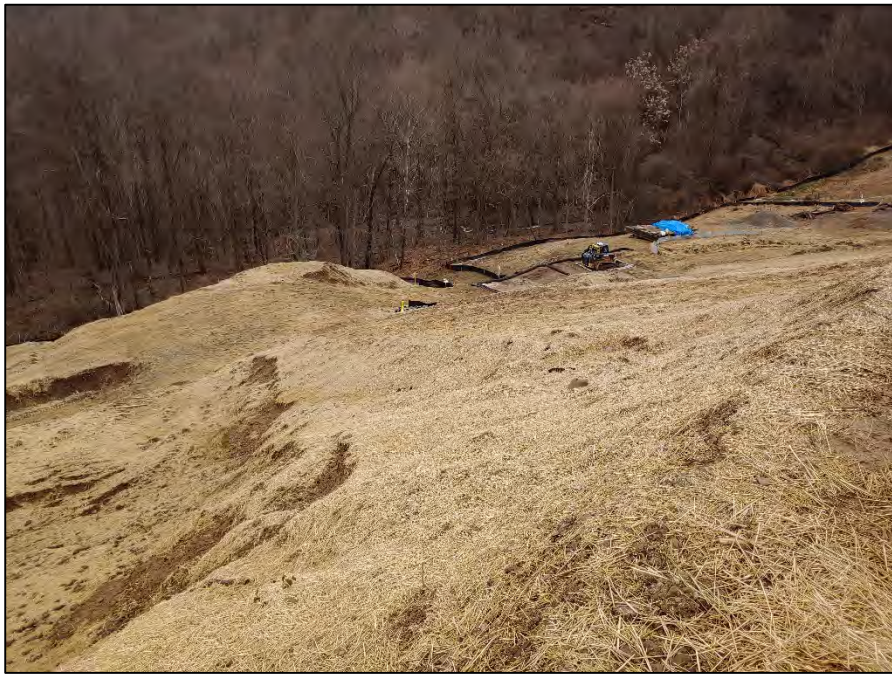
Looking downslope near station 1212+50 along the pipeline alignment
