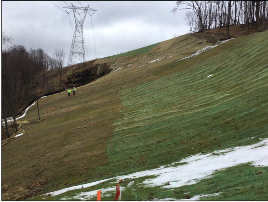
Looking east towards Elkhorn Run 1 near station 868+00
