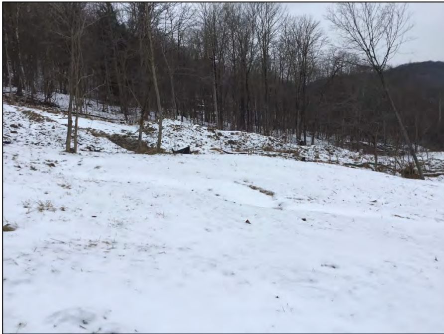
Looking northwest at the landslide near station 1632+00
