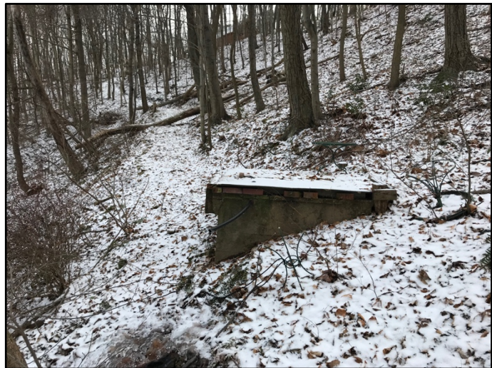
Looking east at a concrete vault on natural slopes north of the pipeline ROW.
