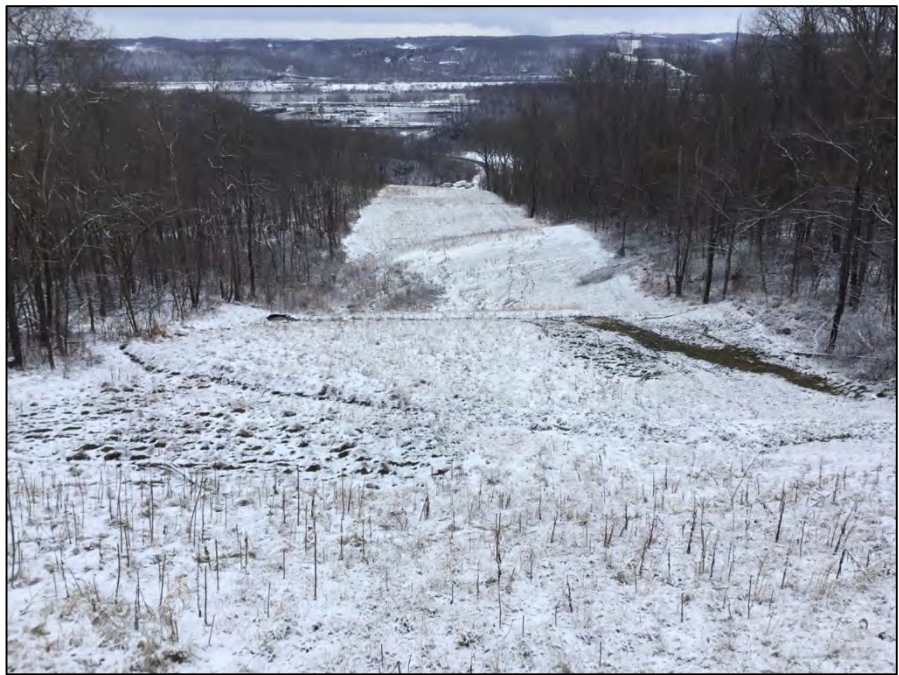
Looking east along the pipeline alignment near station 775+00
