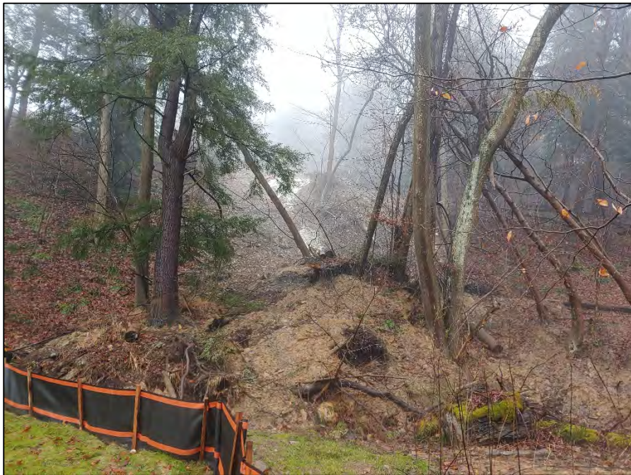
Looking upslope along CIS Elkhorn Run Road near station 888+00
