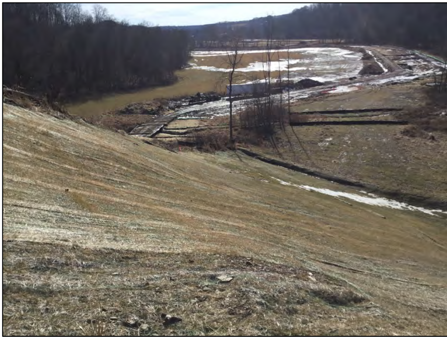
Looking south along the pipeline alignment near station 1737+00
