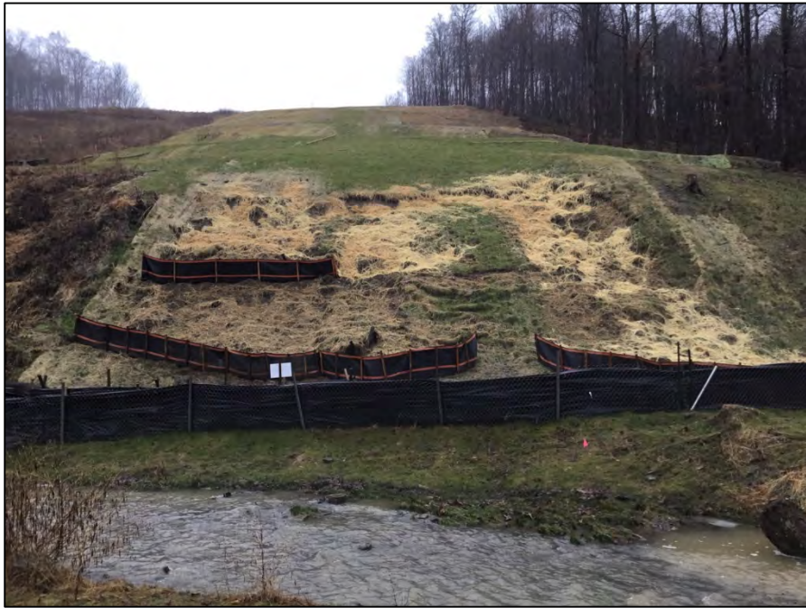
Looking south towards station 1698+00
