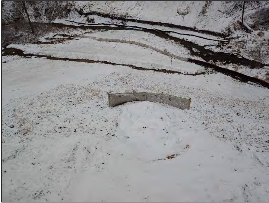
Looking downslope near station 1311+00 along the pipeline alignment
