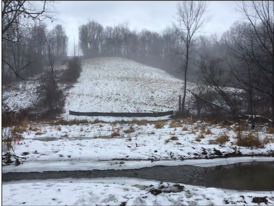
Looking west along the Revolution alignment from near station 655+50
