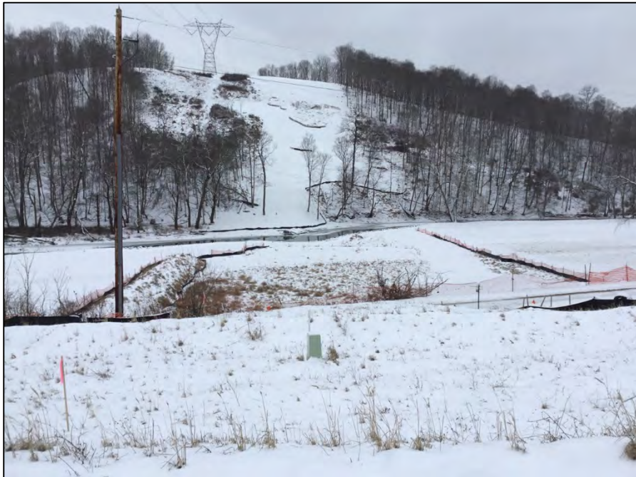
Looking southwest near station 1163+00
