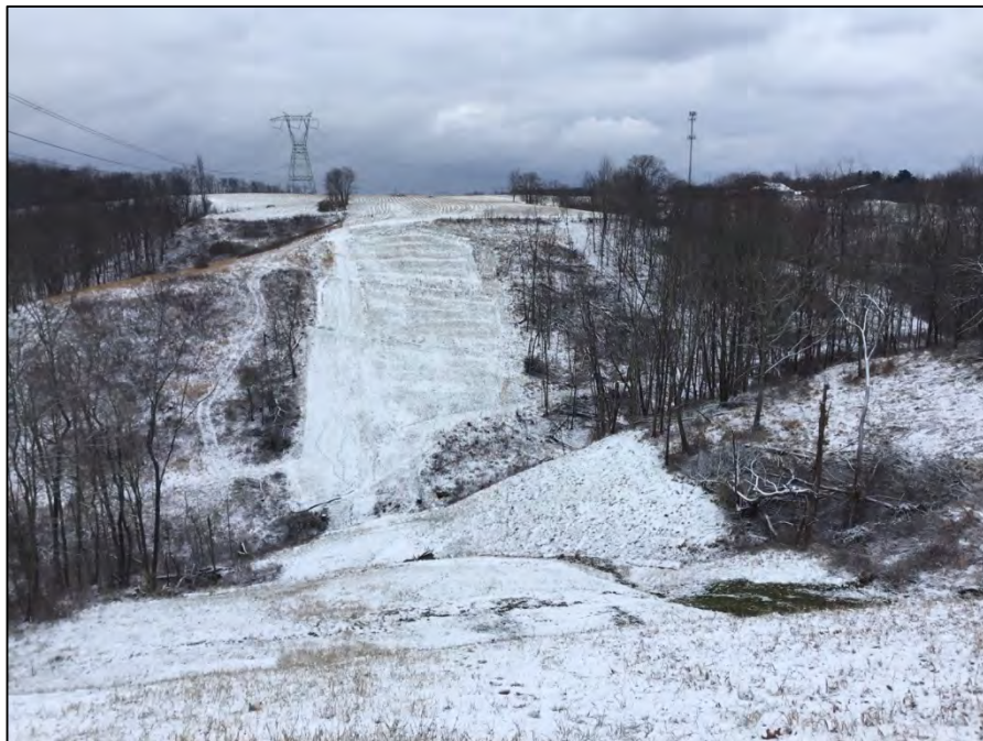
Looking east along the pipeline alignment near station 768+25
