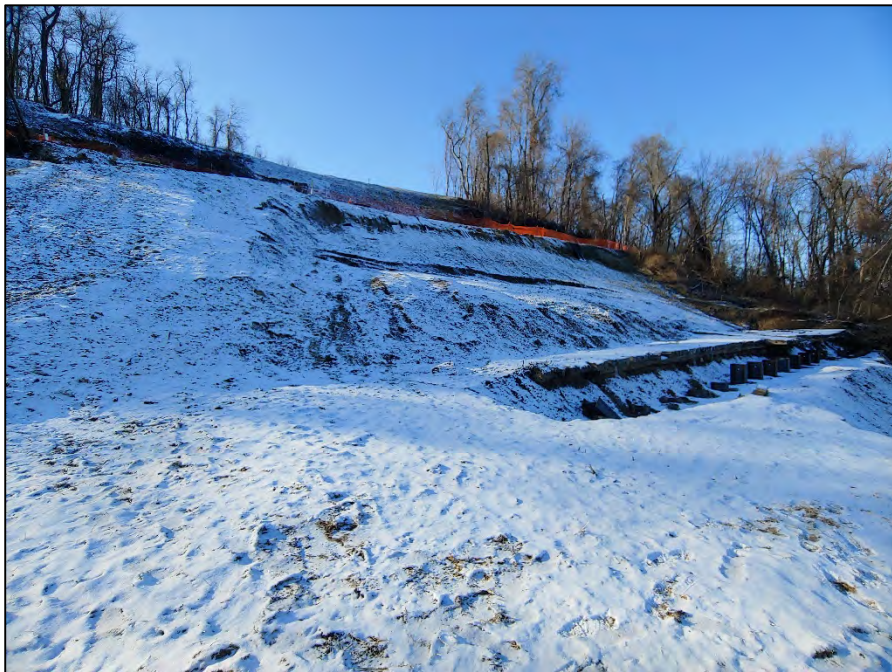
Looking upslope at the soldier pile wall near station 1213+50
