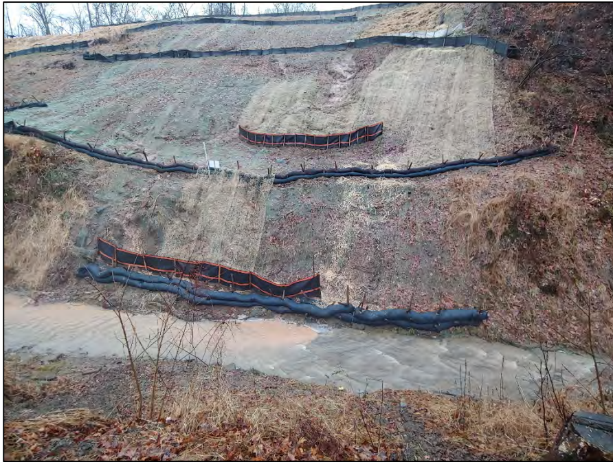
Looking south at station 1495+00
