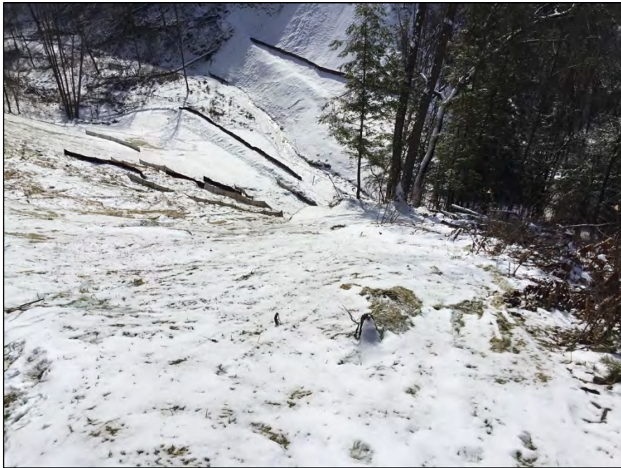
Looking downslope near station 1262+50 along the pipeline alignment
