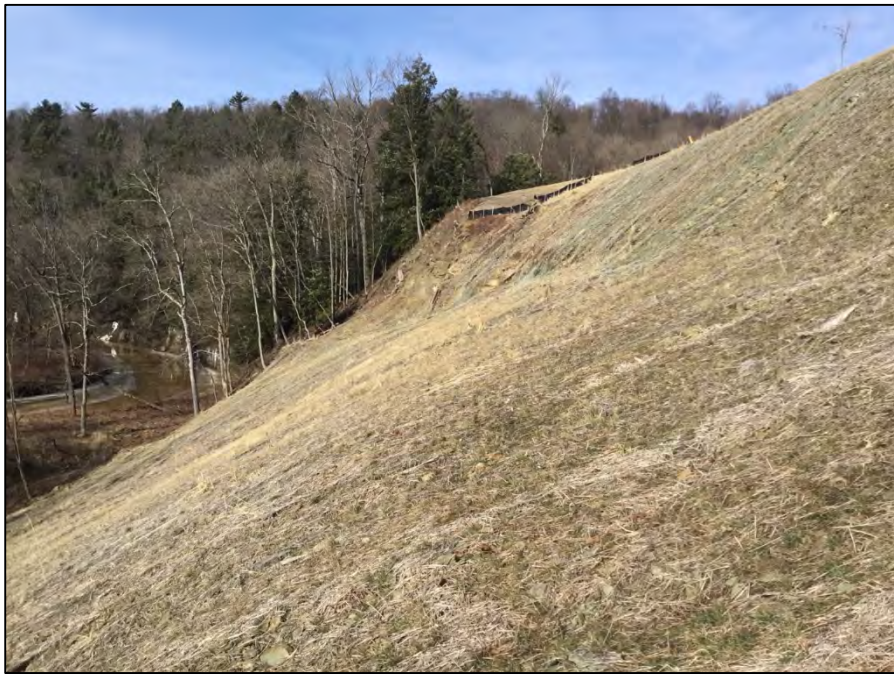
Looking north towards the rock outcrop near station 1737+00
