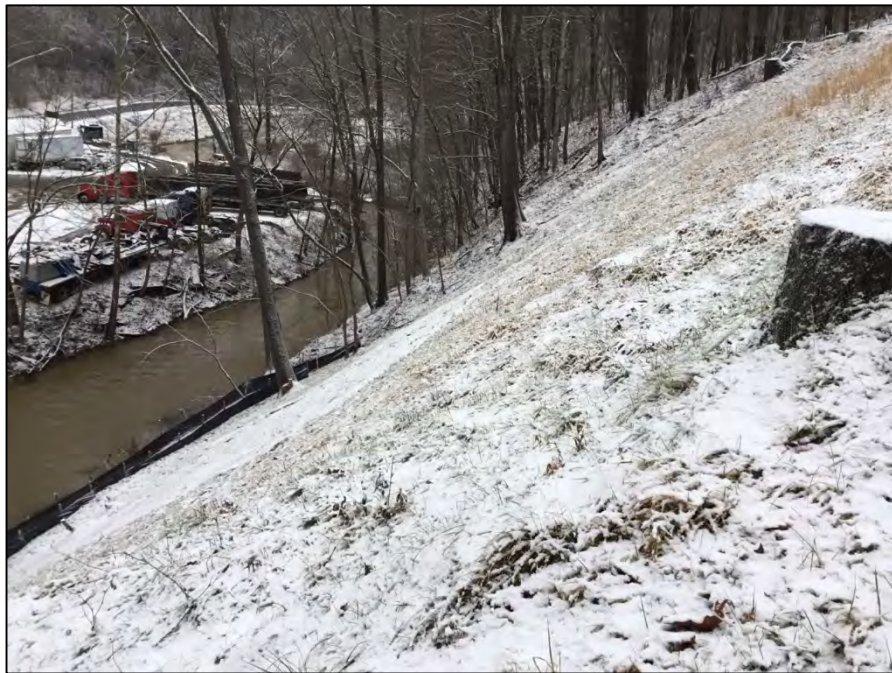
Looking north towards the slope near station 788+00
