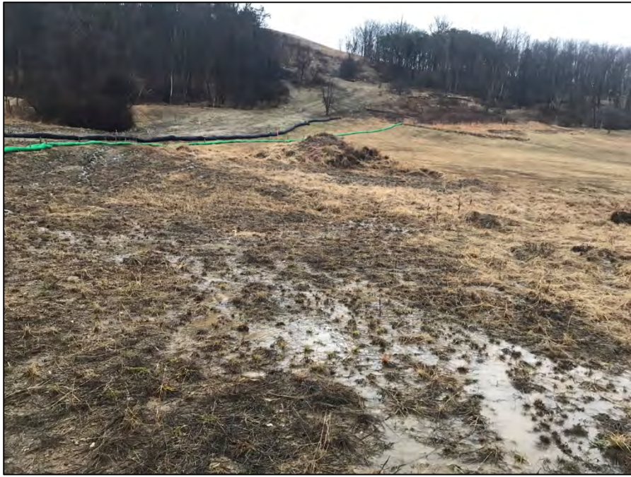
Looking east at groundwater seepage near station 1162+75
