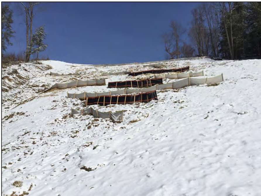
Looking upslope near station 1264+00
