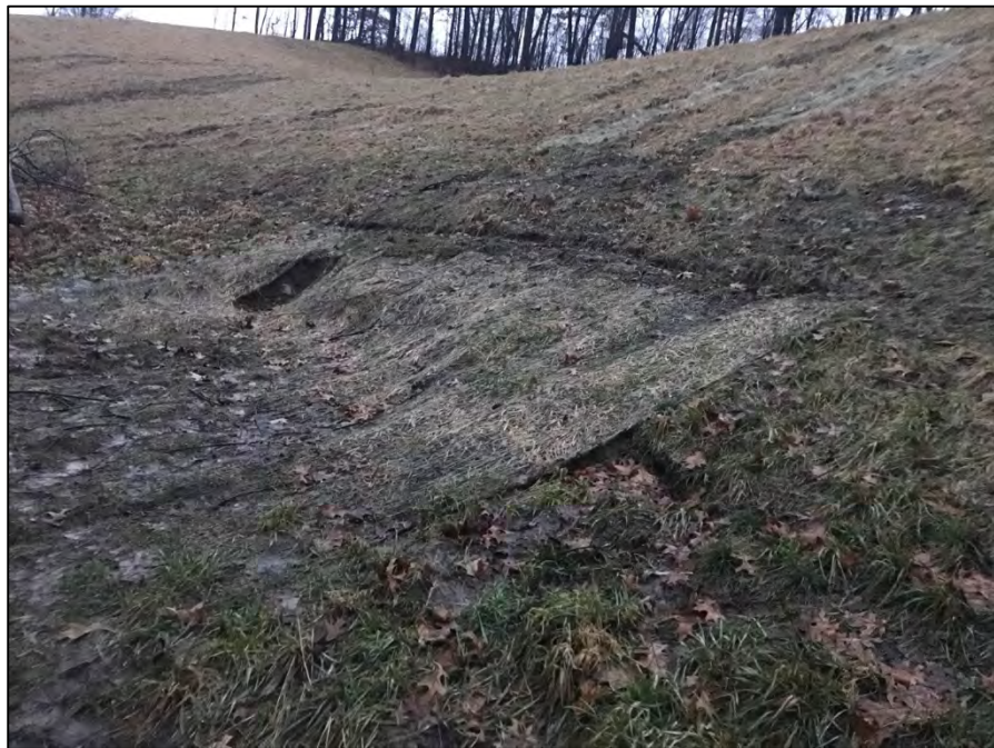
Looking north at the shallow fill failure near station 451+00
