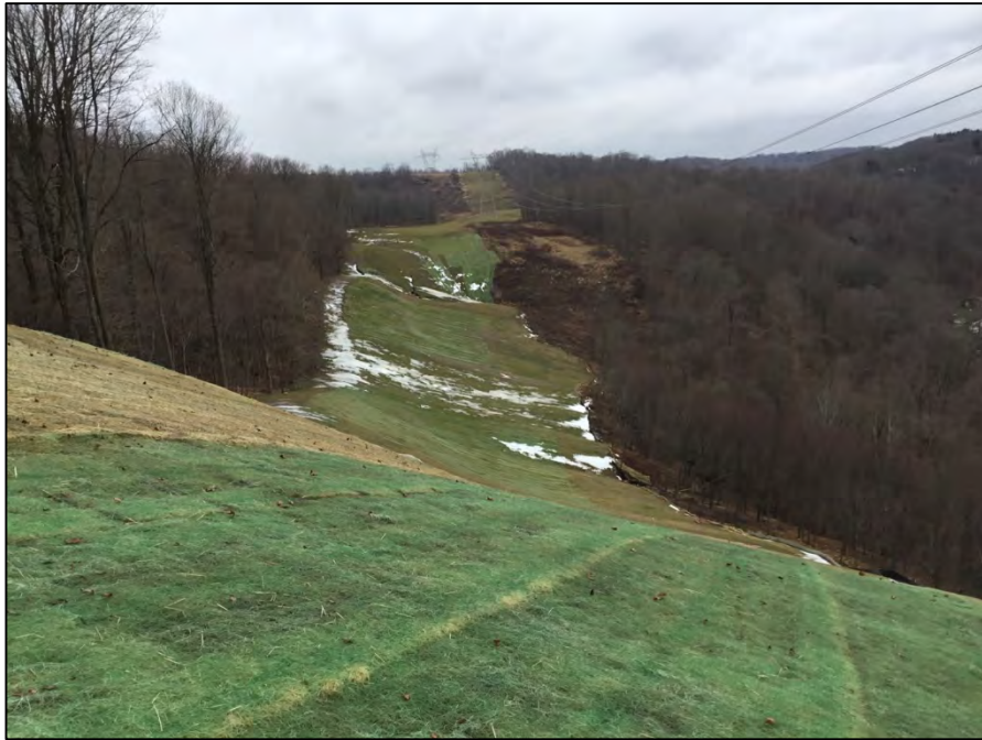
Looking west towards Elkhorn Run 1 near station 864+00
