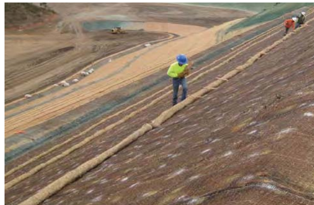
The RollMax TRMs are installed in a one-step operation directly over the prepared seedbed saving time and money and ensuring the highest level of erosion control and vegetation reinforcement.
