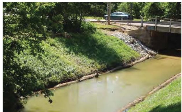
VMax Mats are perfect for pipe outlets, channel bottoms, shoreline transition zones, and other areas subjected to highly turbulent water flows.
