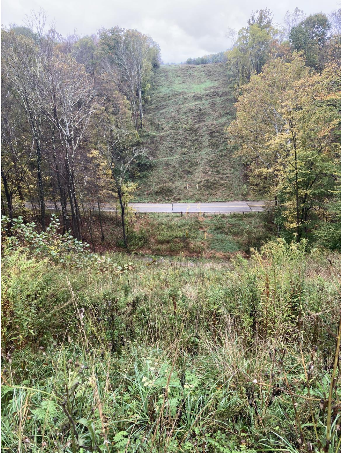
Photograph 7. PA Pipeline ROW looking west from Rippel Road near station 1121+00. Raccoon Run Road is in the middle of the photograph. ROW is stabilized and all temporary erosion controls have been removed. Photograph taken 10/23/2021 by Matt Gordon, ACCD.
