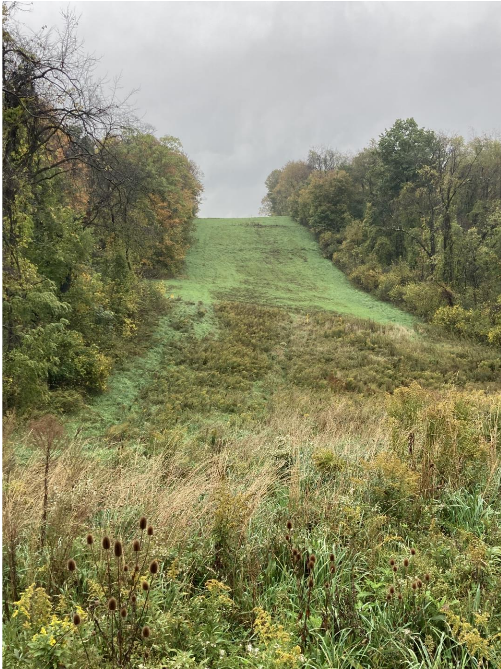
Photograph 4. PA Pipeline ROW looking east near station 1246+50. ROW is stabilized and all temporary erosion controls have been removed. Photograph taken 10/23/2021 by Matt Gordon, ACCD.
