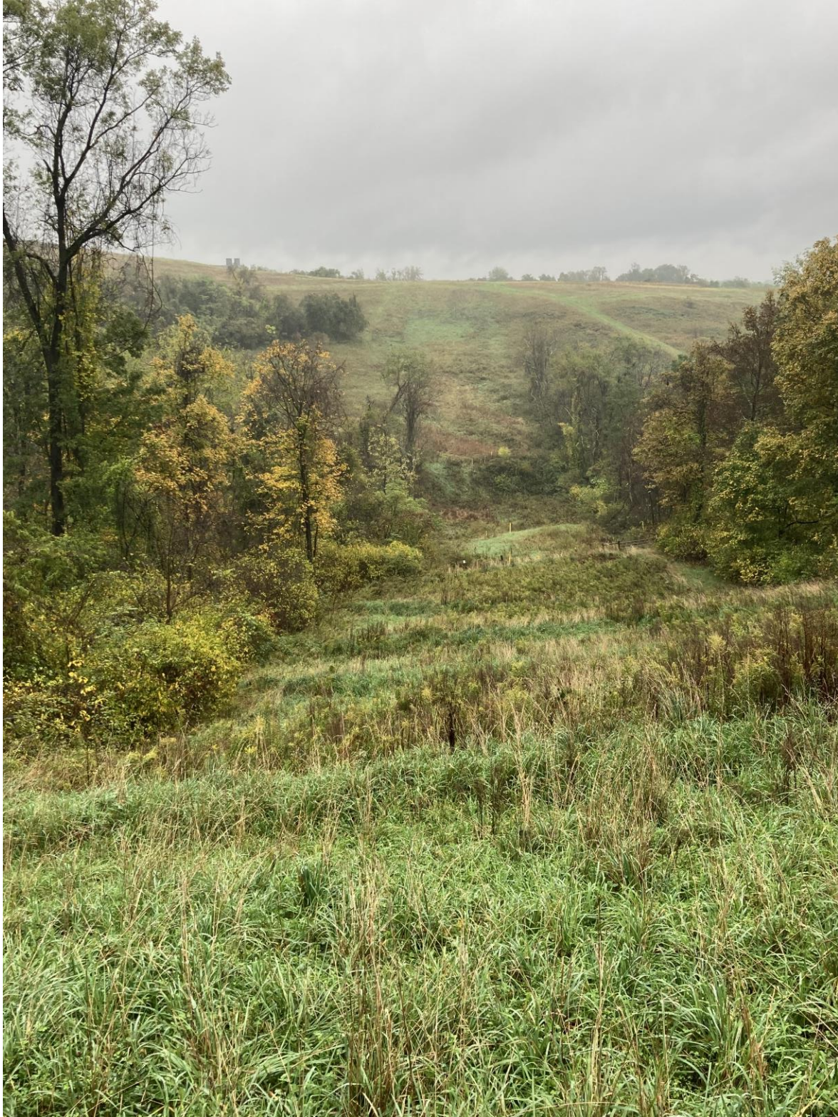
Photograph 5. PA Pipeline ROW near 1252+00 looking east. ROW is stabilized and all temporary erosion controls have been removed. Photograph taken 10/23/2021 by Matt Gordon, ACCD.
