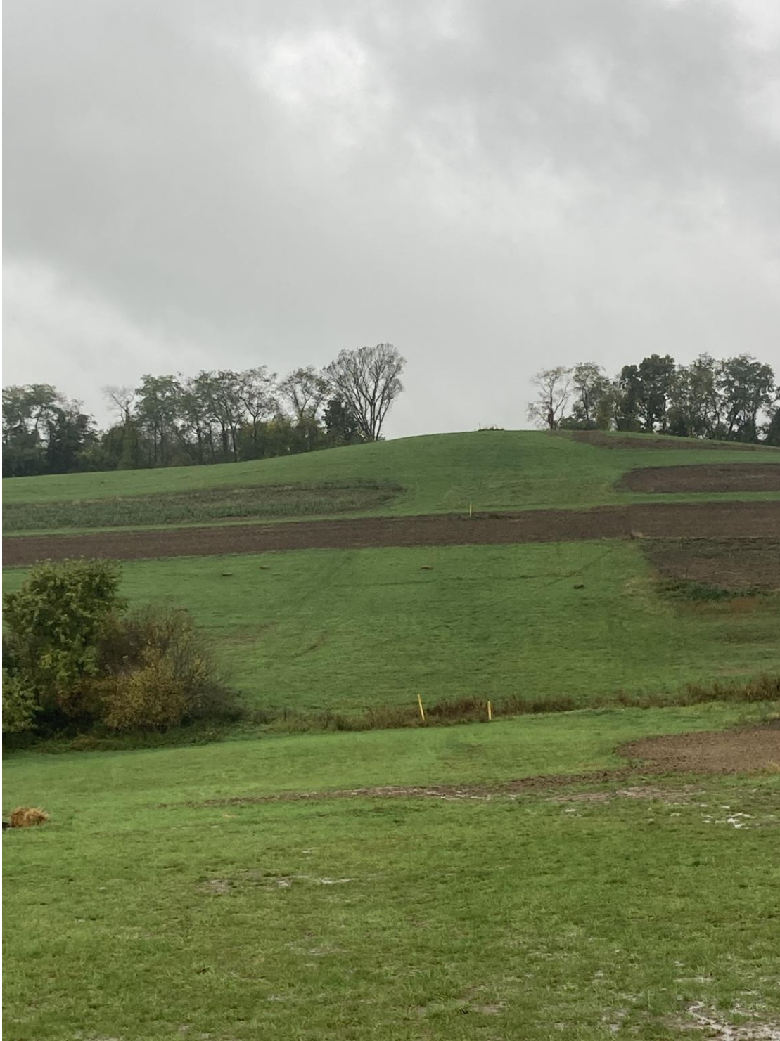
Photograph 2. PA Pipeline ROW looking west near station 1222+00 from Williamsport Road. The property owner has been farming over ROW. Temporary controls have been removed and ROW is stabilized outside of farming activities. Photograph taken 10/23/2021 by Matt Gordon, ACCD.
