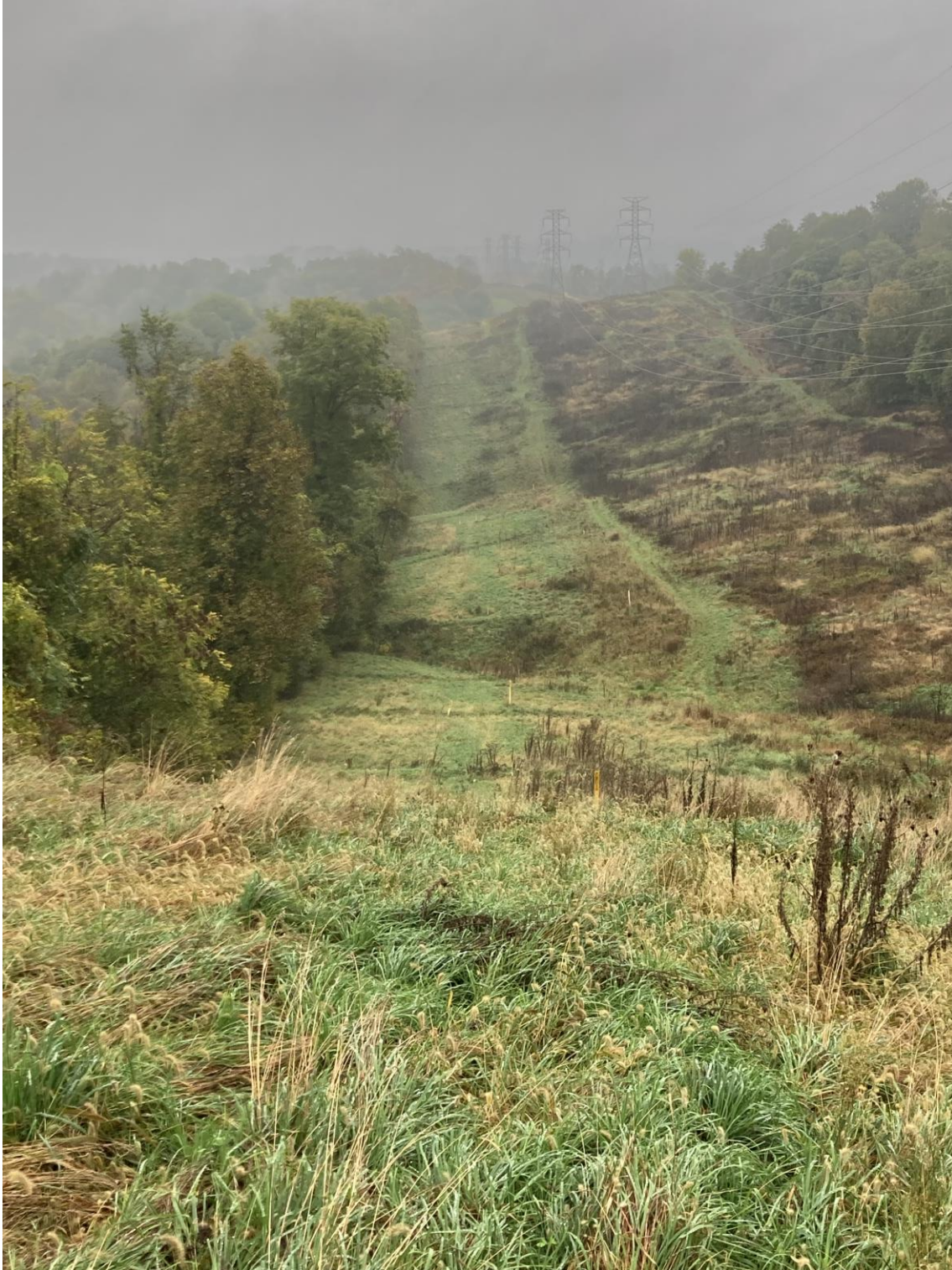
Photograph 1. PA Pipeline ROW looking east near station 1462+50 into Westmoreland County. ROW is stabilized and all temporary erosion controls have been removed. Photograph taken 10/23/2021 by Matt Gordon, ACCD.
