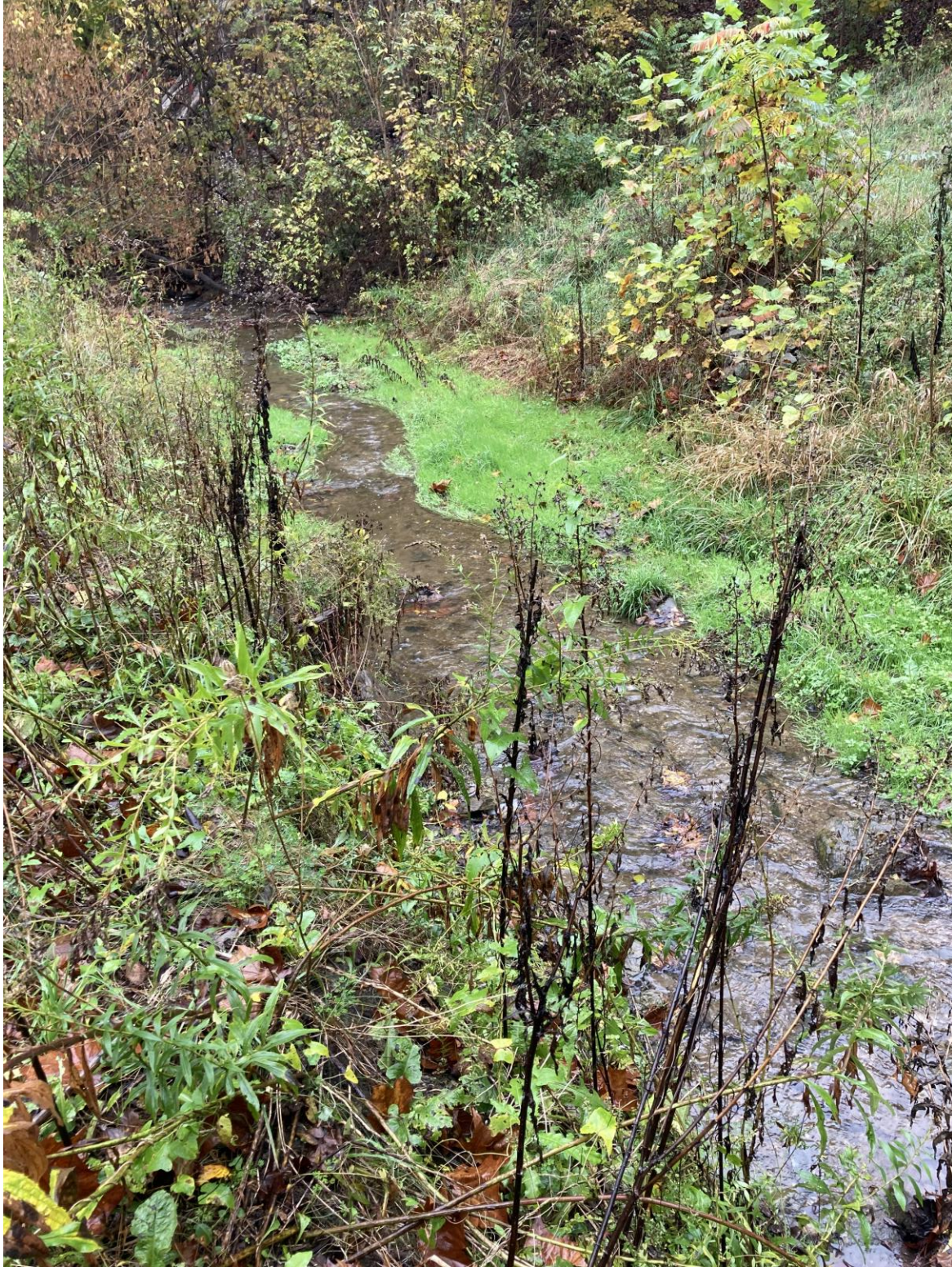
Photograph 6. PA Pipeline ROW near Pangburn Hollow Road crossing of Perry Mill Run near station 1184+50. ROW is stabilized and all temporary erosion controls have been removed. Photograph taken 10/23/2021 by Matt Gordon, ACCD.
