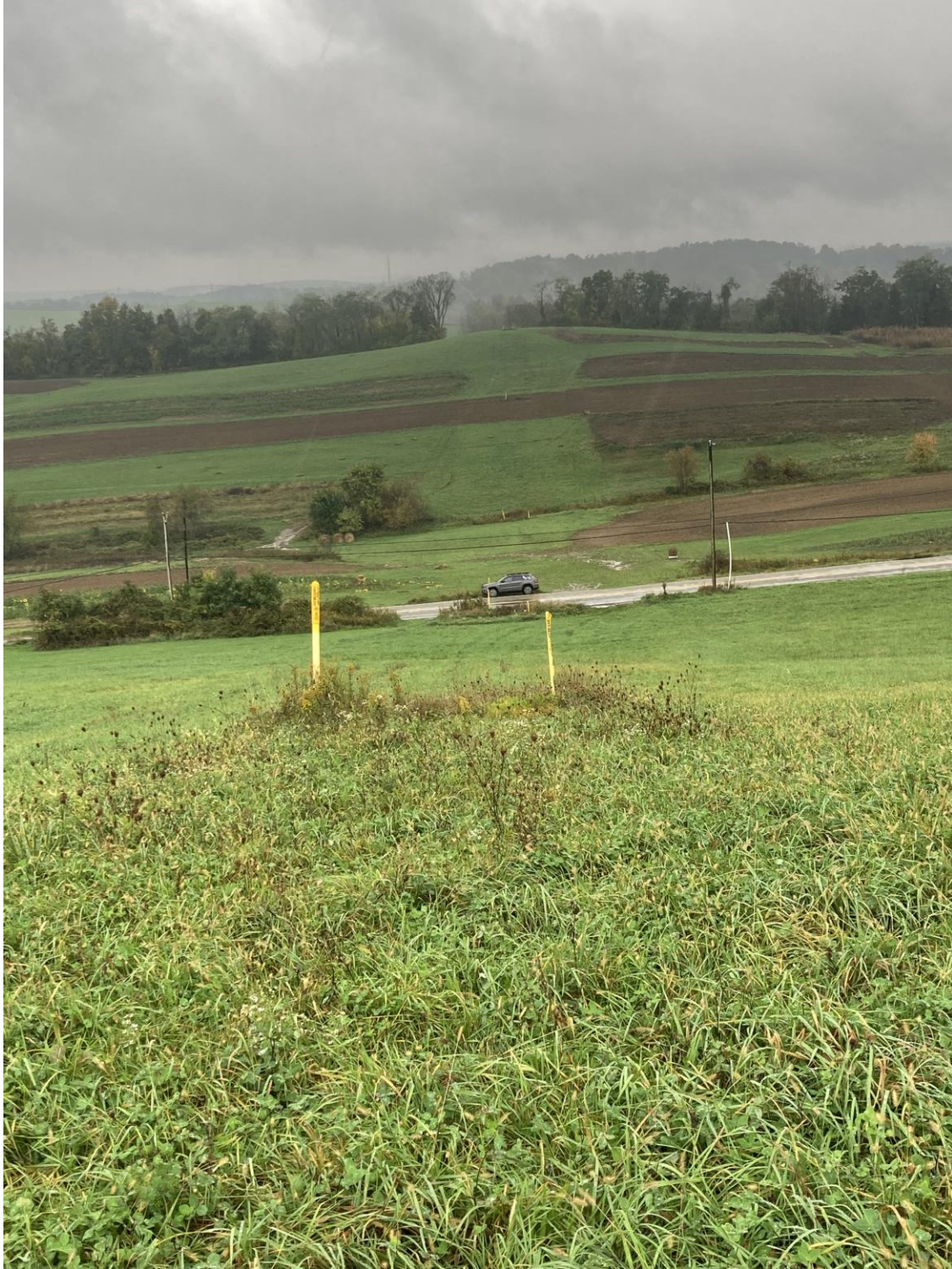
Photograph 3. PA Pipeline ROW looking west near station 1226+00. ROW is stabilized and all temporary erosion controls have been removed. Photograph taken 10/23/2021 by Matt Gordon, ACCD.
