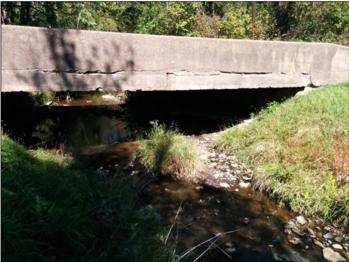
Ullom Road Bridge Looking Upstream on Westland Run
