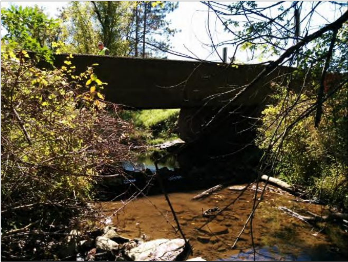
Ullom Road Bridge Looking Downstream on Westland Run
