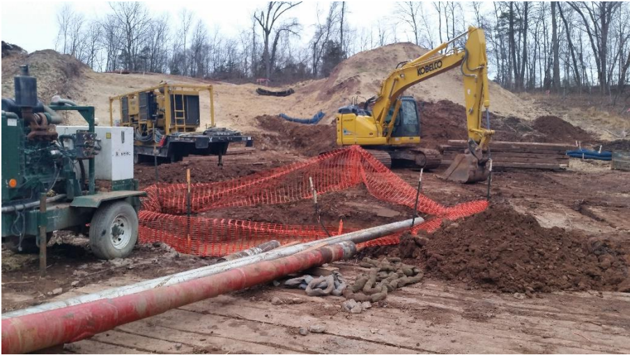
Excavation West Side of HDD alignment.
