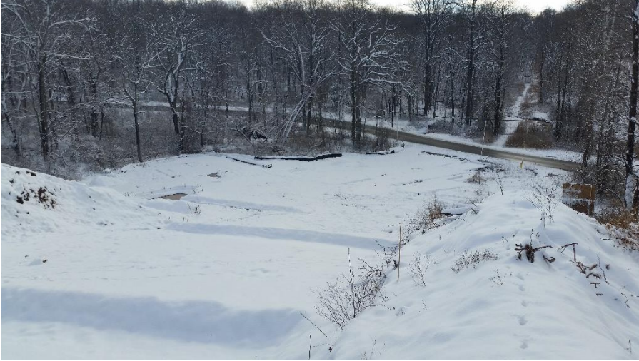
February 18, 2018 Looking East along the HDD route.
