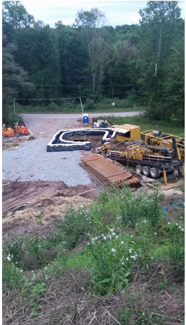
September 22, 2018 Erosion and Sediment (E&S) Controls are increased around the drilling pit.
