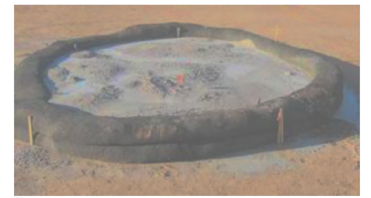
FIGURE 3.18 Typical Compost Sock Washout Installation
