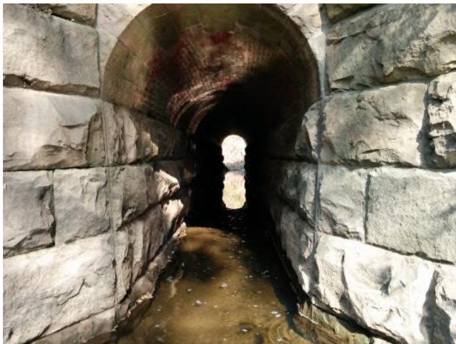
Photo 1: Railroad Culvert Facing Upstream
