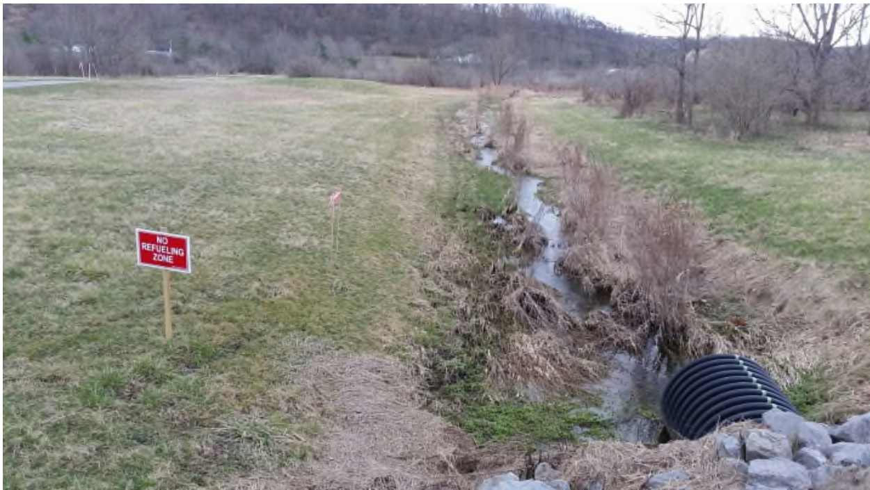
Photo 2: E. Loop Road Culvert Inlet Looking South
