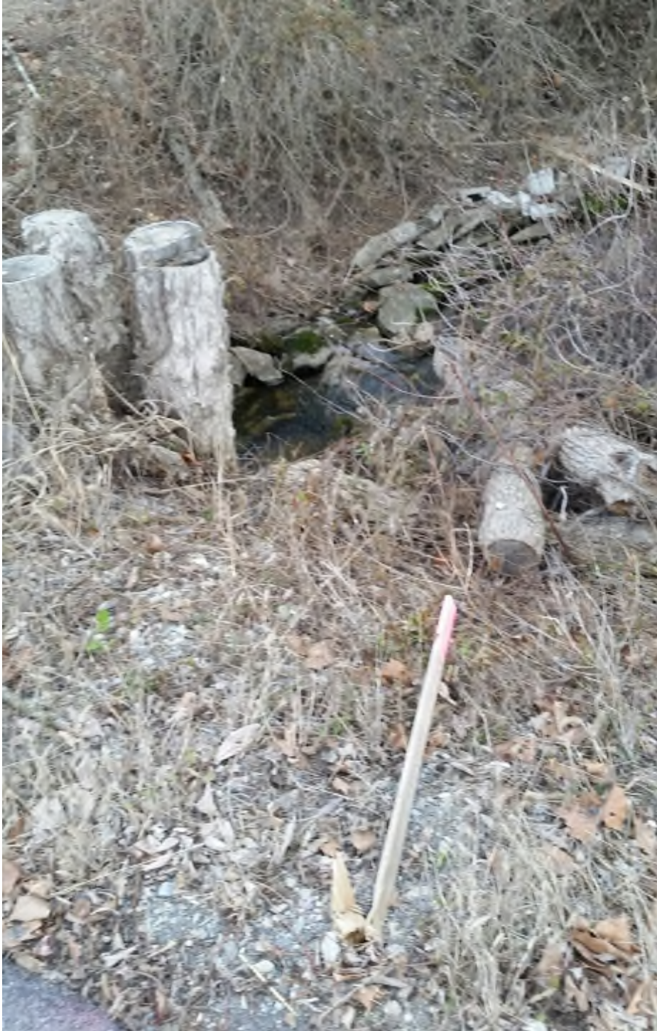
Photo 3: E. Loop Rd. Culvert Outlet Looking North
