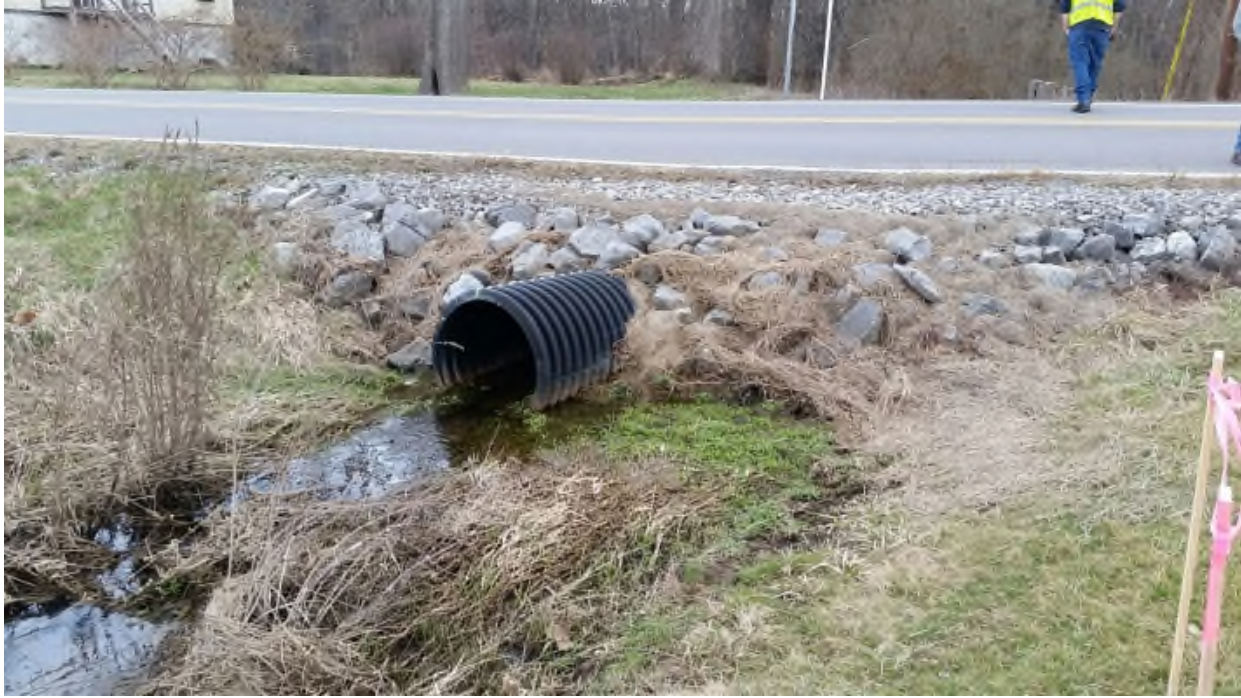
Photo 1: E. Loop Road Culvert Inlet Looking North
