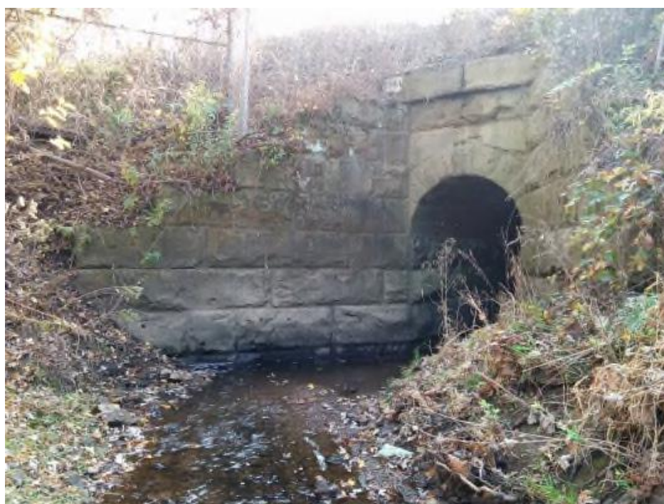
Photo 2: Railroad Culvert Facing Downstream
