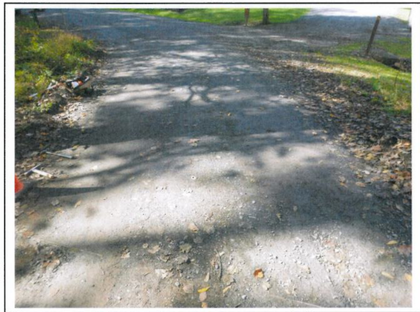
Photo No. 18: Near Approach Condition
