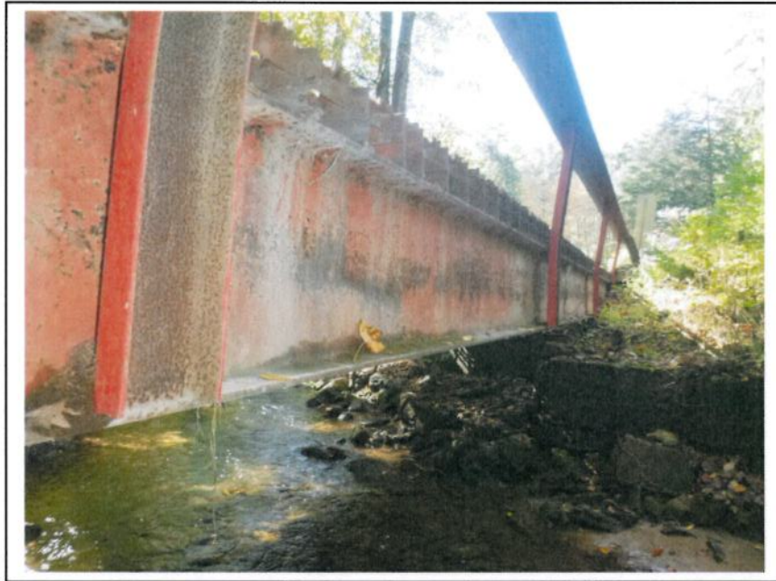
Photo No. 23: Beam 1 Fascia
