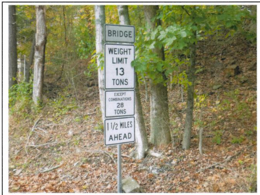
Photo No. 10: Far Advanced Weight Posting Sign
