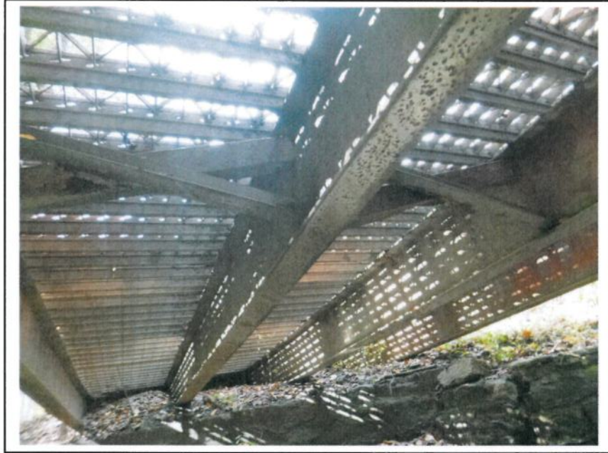
Photo No. 21: Typical Underside
