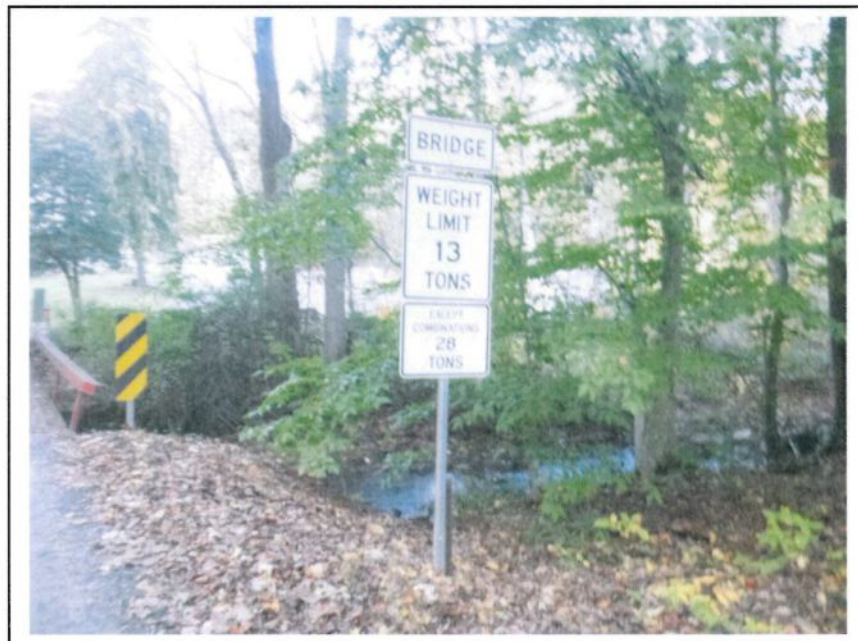
Photo No. 12: Far Weight Limit Sign
