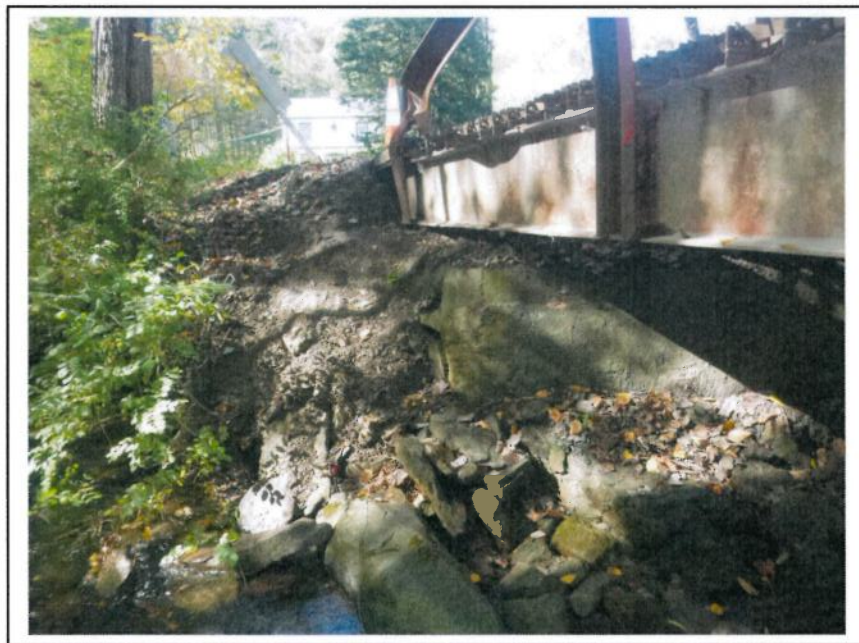
Photo No. 34: Near Right Wing Elevation
