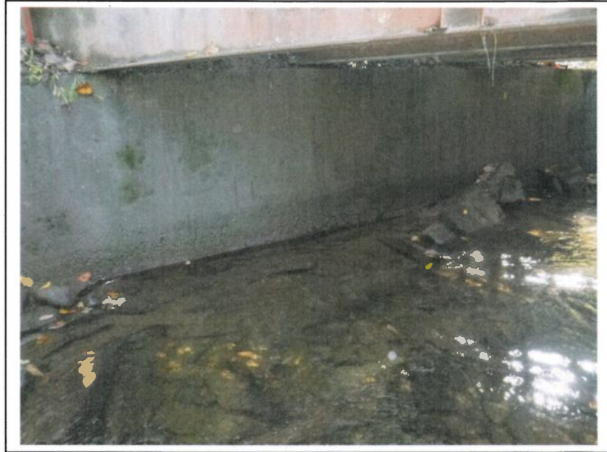
Photo No. 35: Far Abutment Elevation
