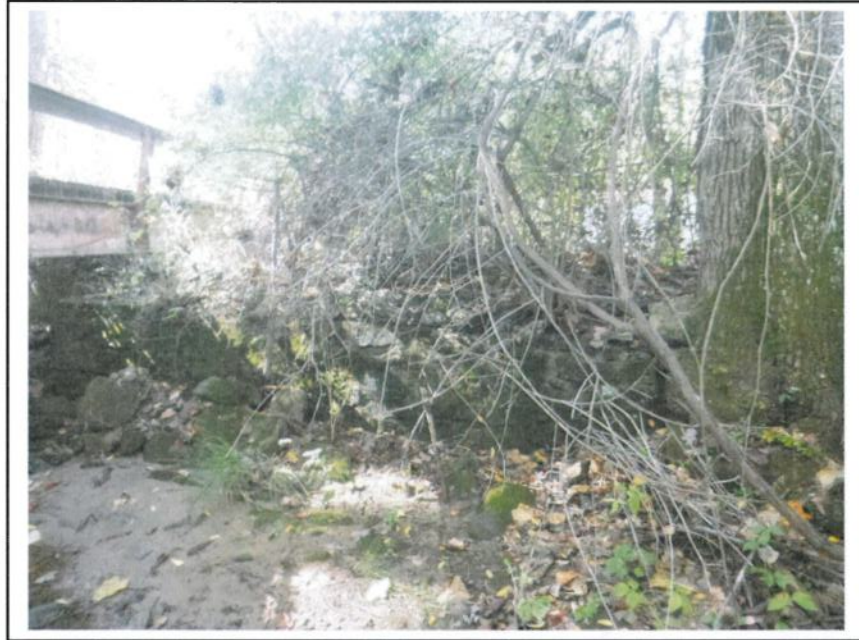
Photo No. 33: Near Left Wing Elevation
