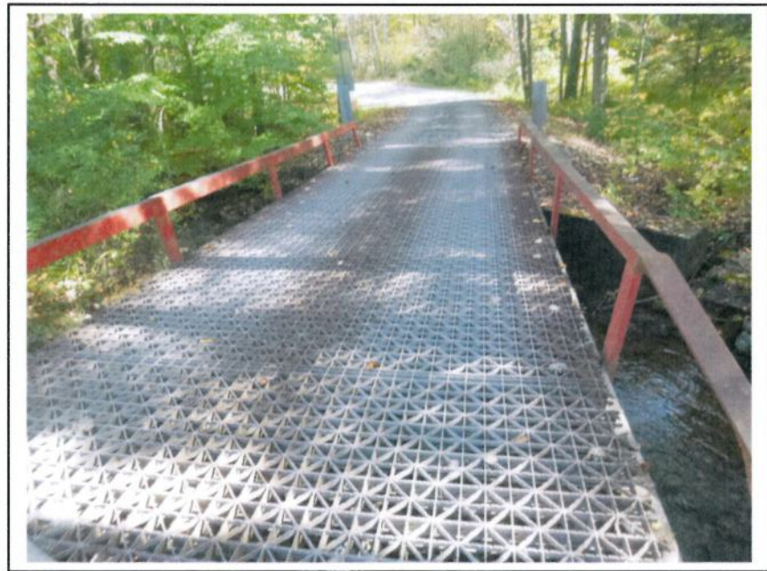
Photo No. 20: Typical Deck Condition
