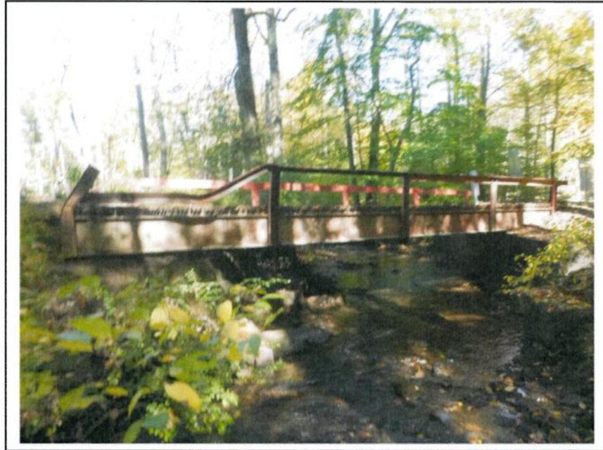
Photo No. 5: Upstream Elevation
