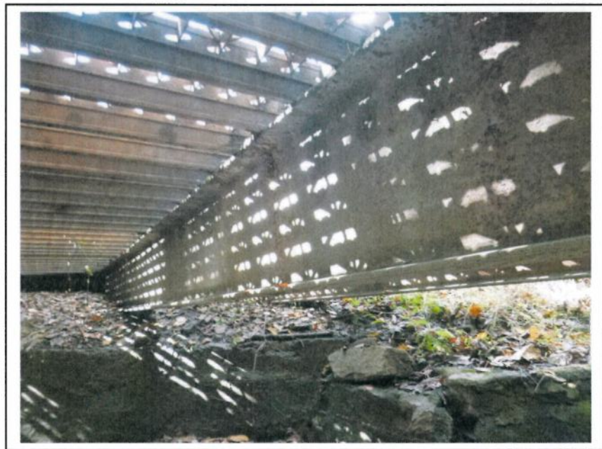
Photo No. 24: Beam 2 Web
