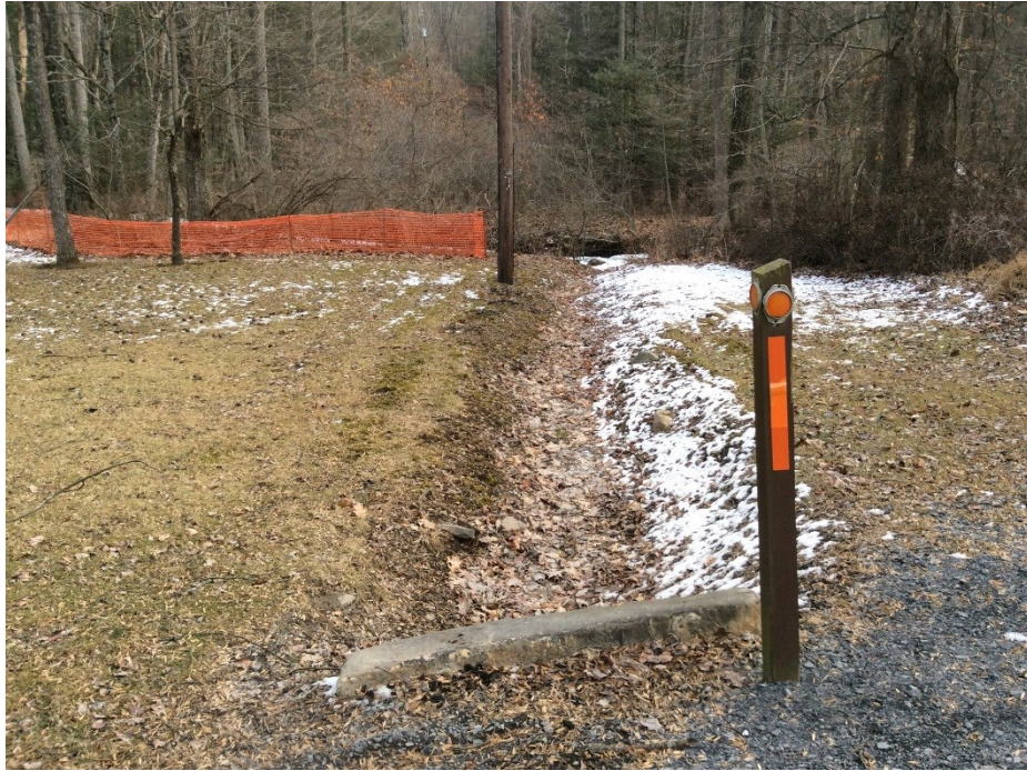
Photograph 3. S-JA2. Facing east.
