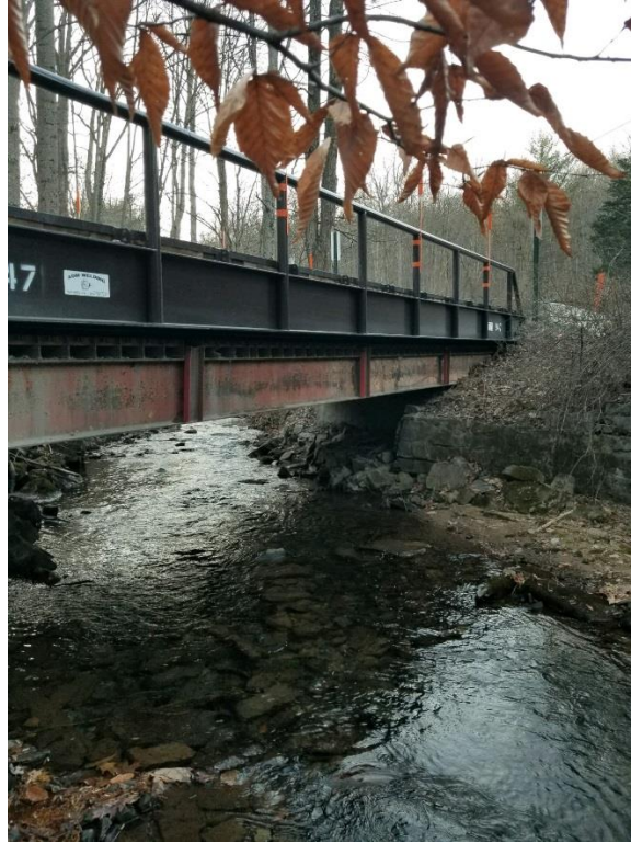
Photo 1 – 12/18/2017 – Looking southwest at bridge.
