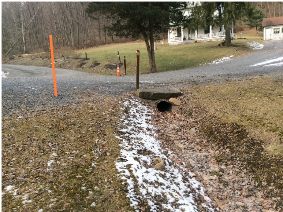
Photograph 4. S-JA2 Facing west.
