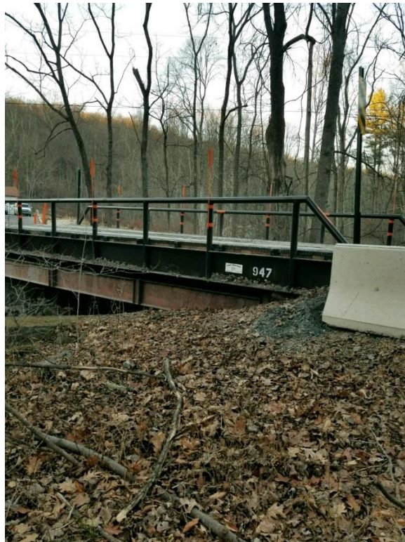
Photo 4 – 12/18/2017 – Looking southeast at bridge.
