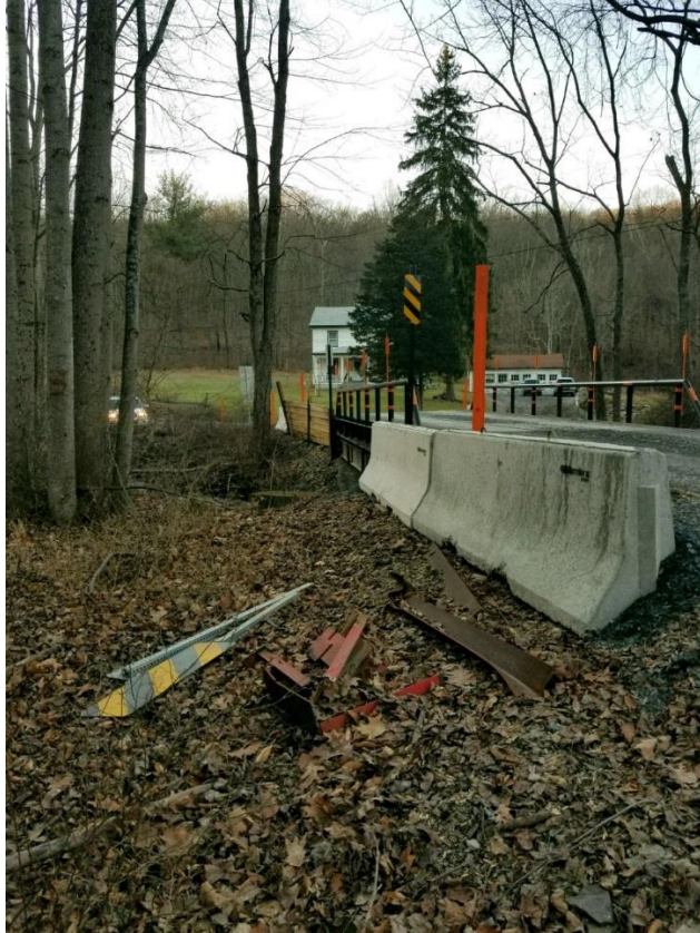
Photo 5 – 12/18/2017 – Looking northwest across bridge.
