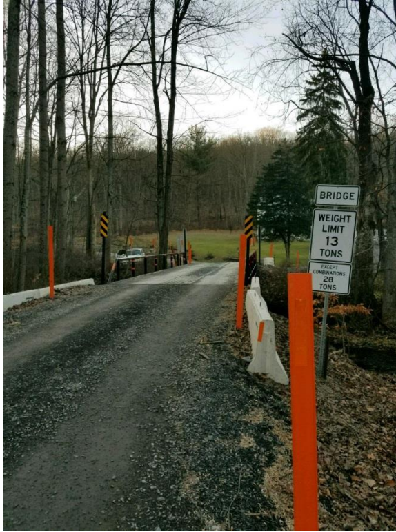
Photo 3 – 12/18/2017 – Looking west across bridge.
