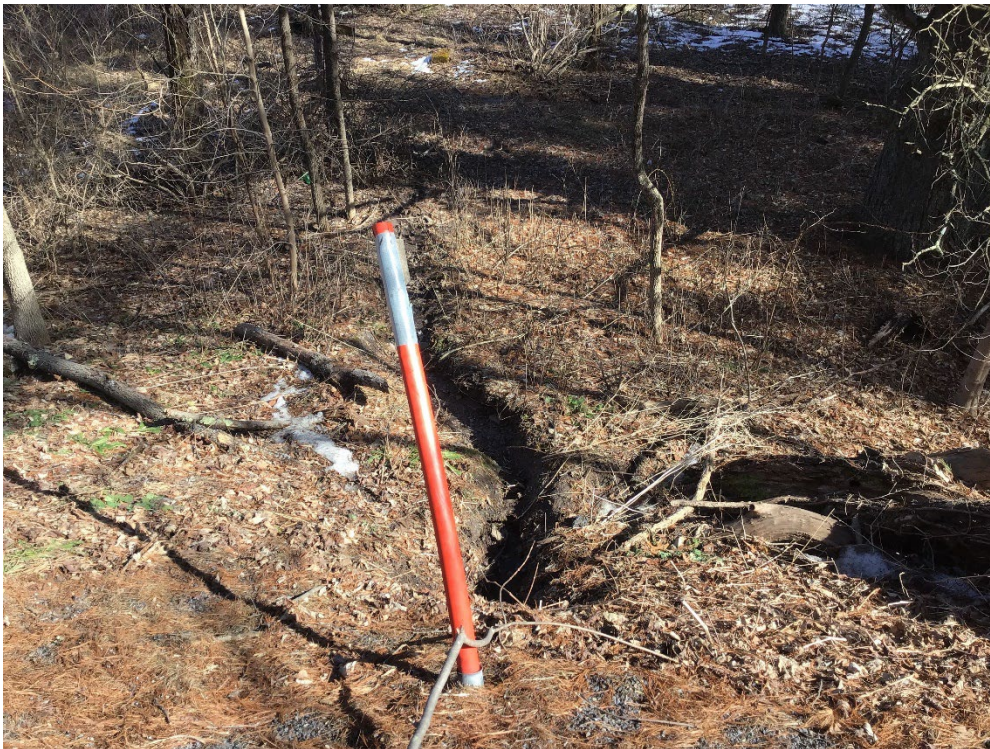
Photo 7: Existing Area Downgradient of PennDOT Culvert
