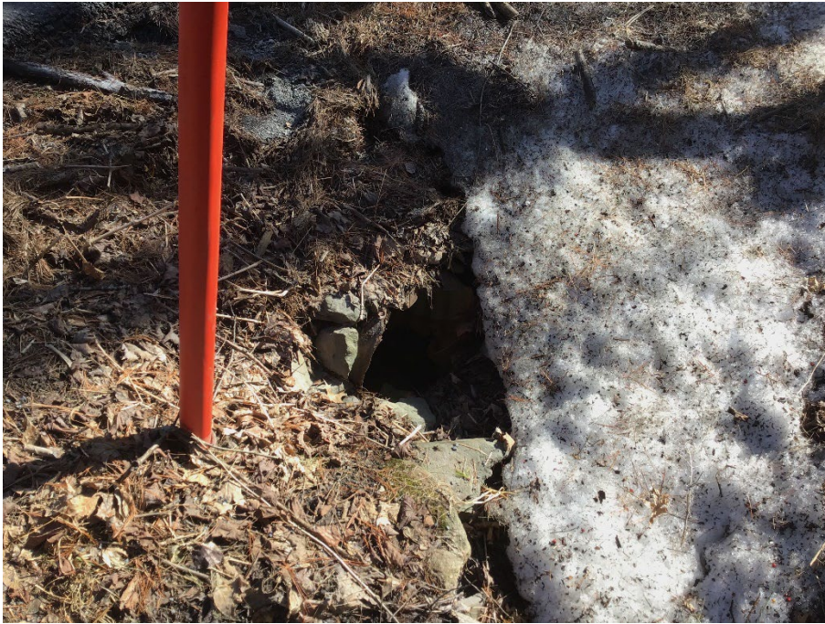
Photo 6: Existing PennDOT Culvert Inlet
