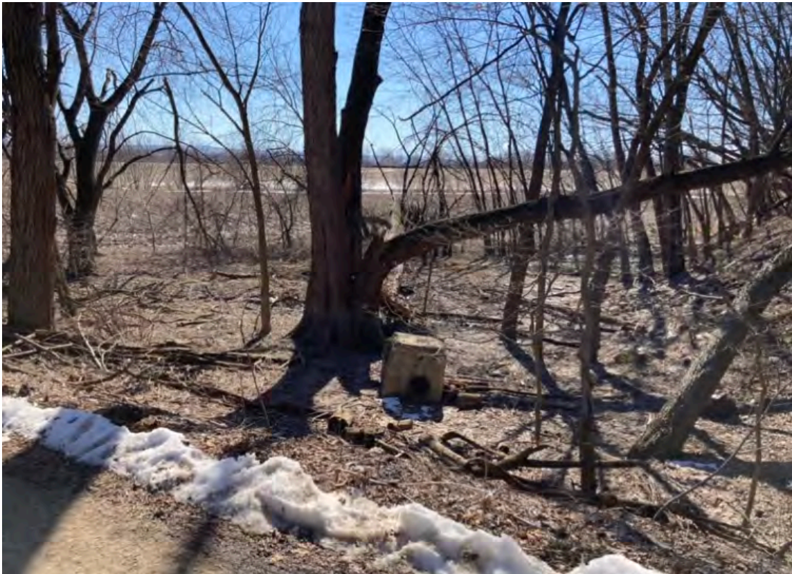
Photo 1: Existing Area at Proposed Rip-Rap Apron
