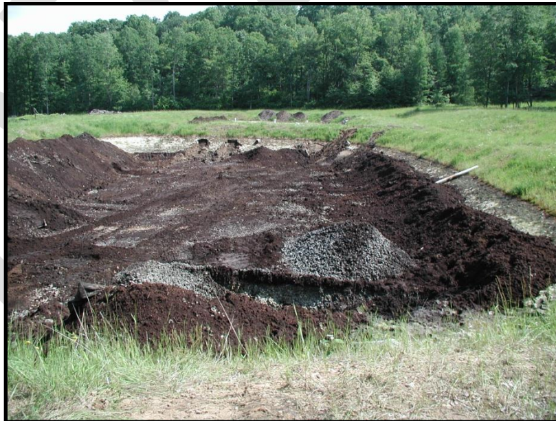
Figure 7.7. The compost layer being placed on top of the limestone layer in a VFP
