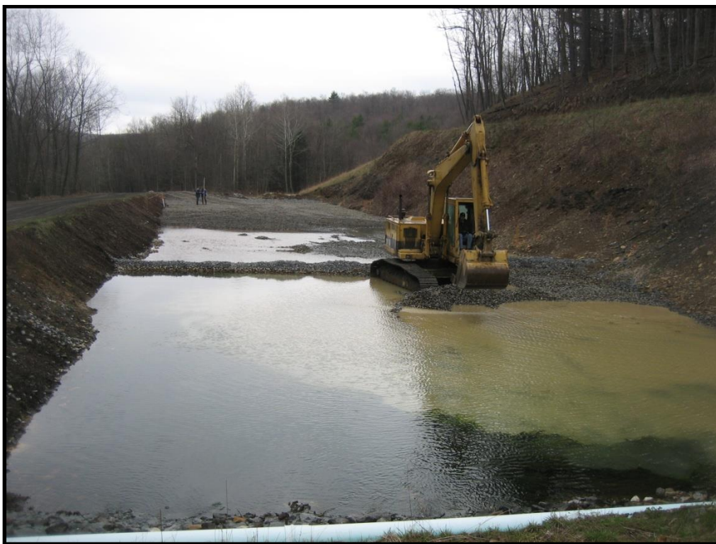
Figure 7.14. Agitation using an excavator to break up precipitate and reestablish flow in a clogged section of a RLB
