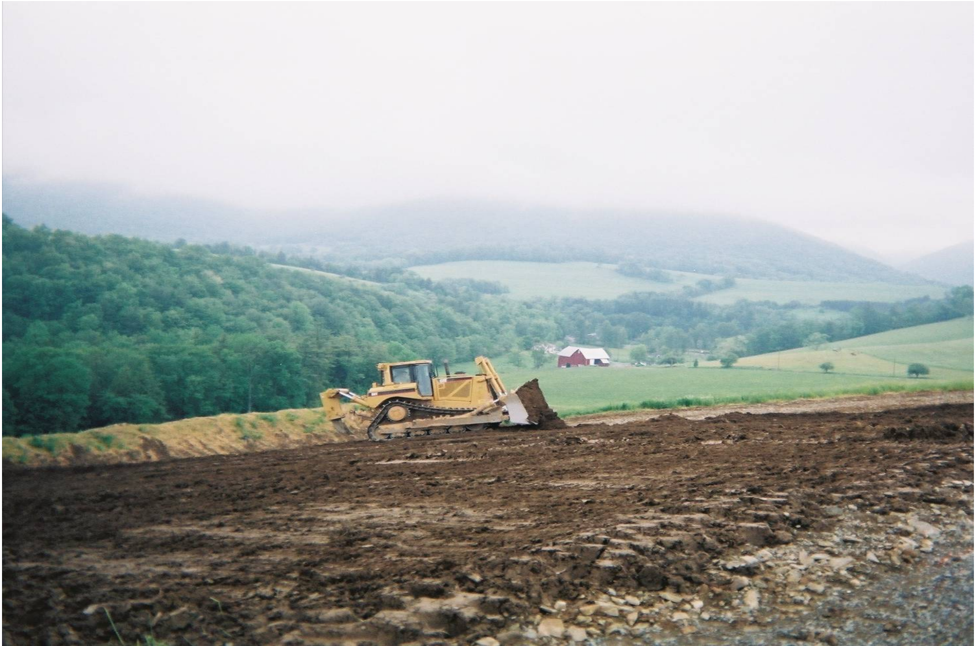
Topsoil being spread
