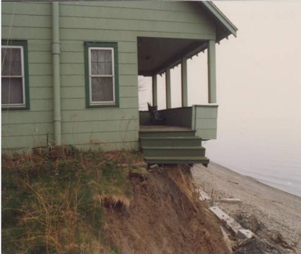
Residence undercut by wave damage and bluff recession in the Woodmere Sub-division, North East Township (1987) Structure removed via NFIP claim (Upton/Jones)
