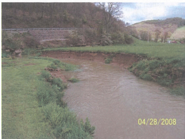
HQ 9 Upstream Reach (downstream)
