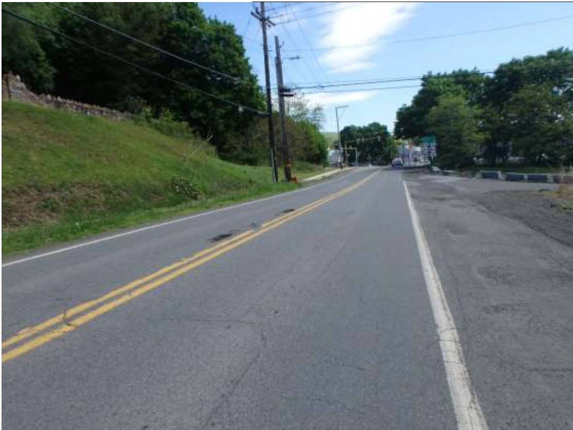
Direction / Road: EB Hancock Street Approach / Departure: Approach Distance: 200 feet
