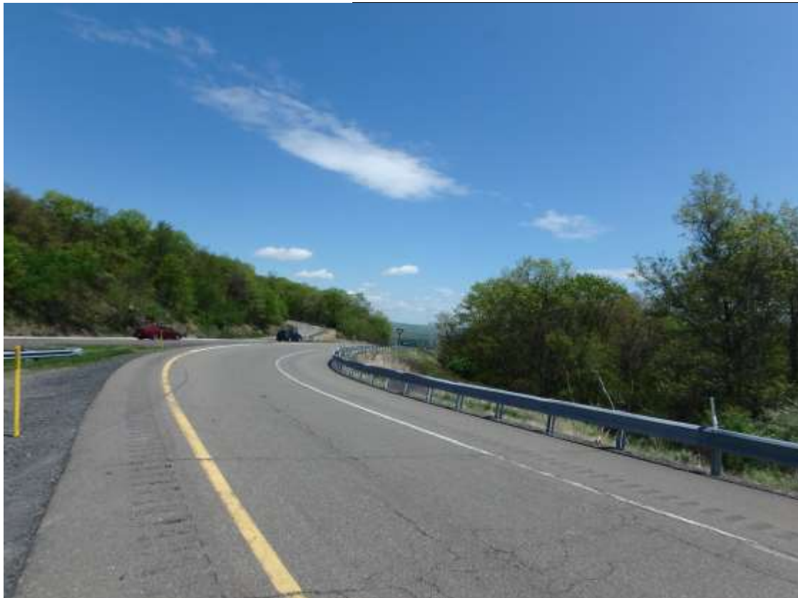
Direction / Road: EB I-81 NB on/off-ramps Approach / Departure: Approach Distance: 200 feet
