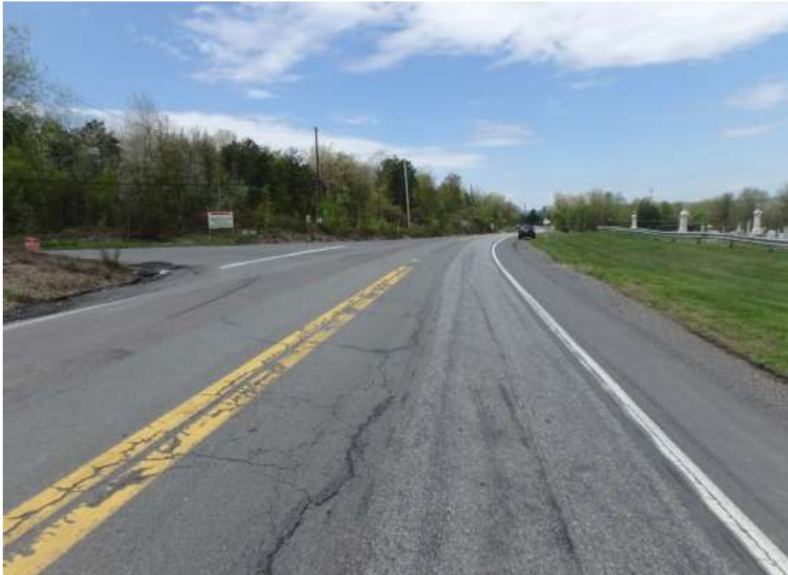
Direction / Road: WB Morea Road Approach / Departure: Approach Distance: 50 feet
