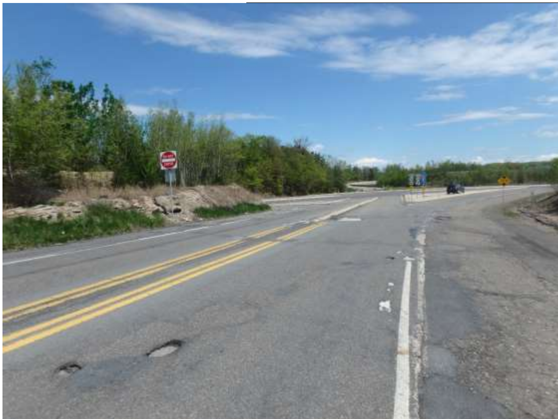
Direction / Road: EB I-81 SB on/off-ramps Approach / Departure: Approach Distance: 200 feet
