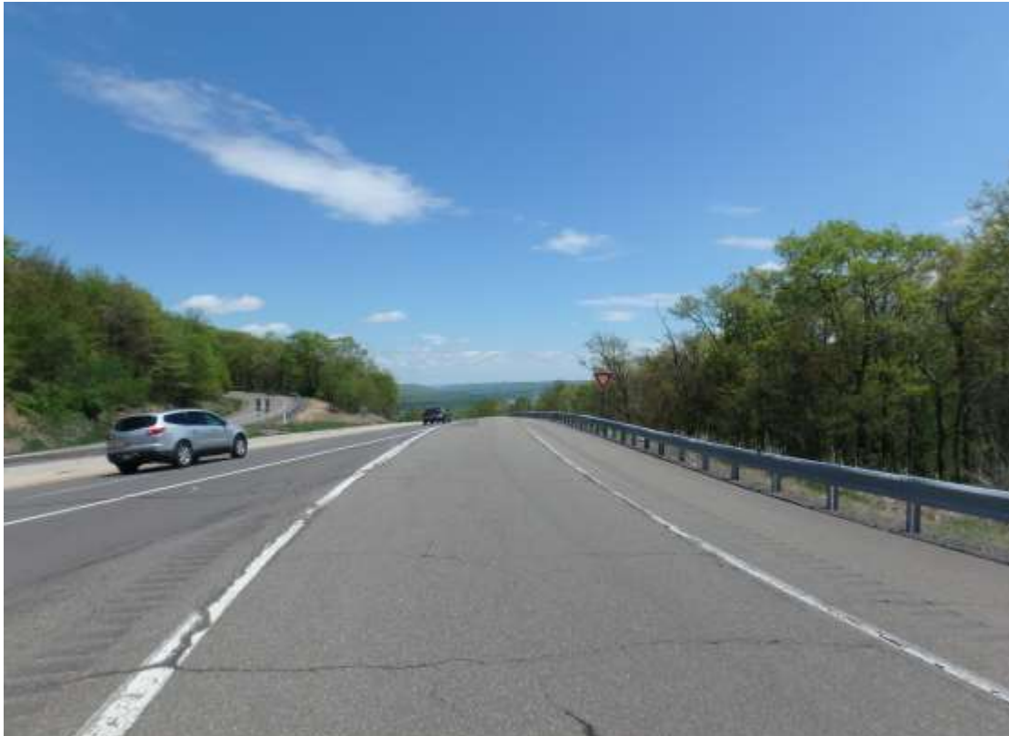
Direction / Road: EB I-81 NB on/off-ramps Approach / Departure: Approach Distance: 50 feet
