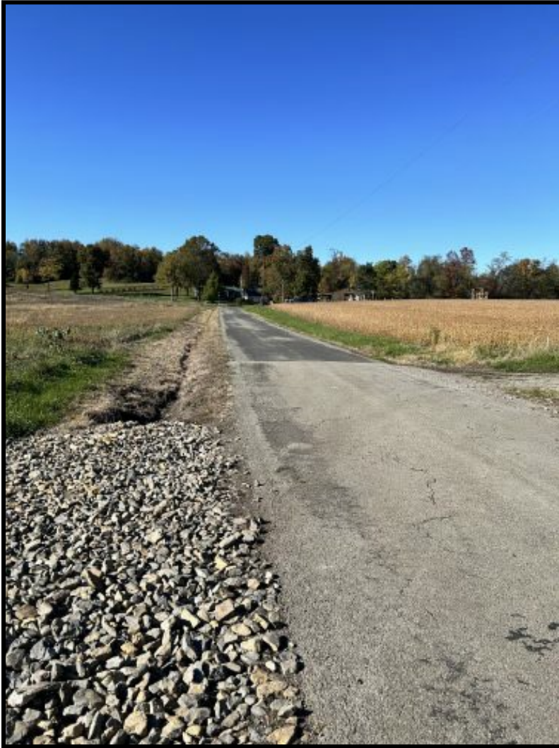
Photograph 9 –Road crossing at approximate Station 117+00.
