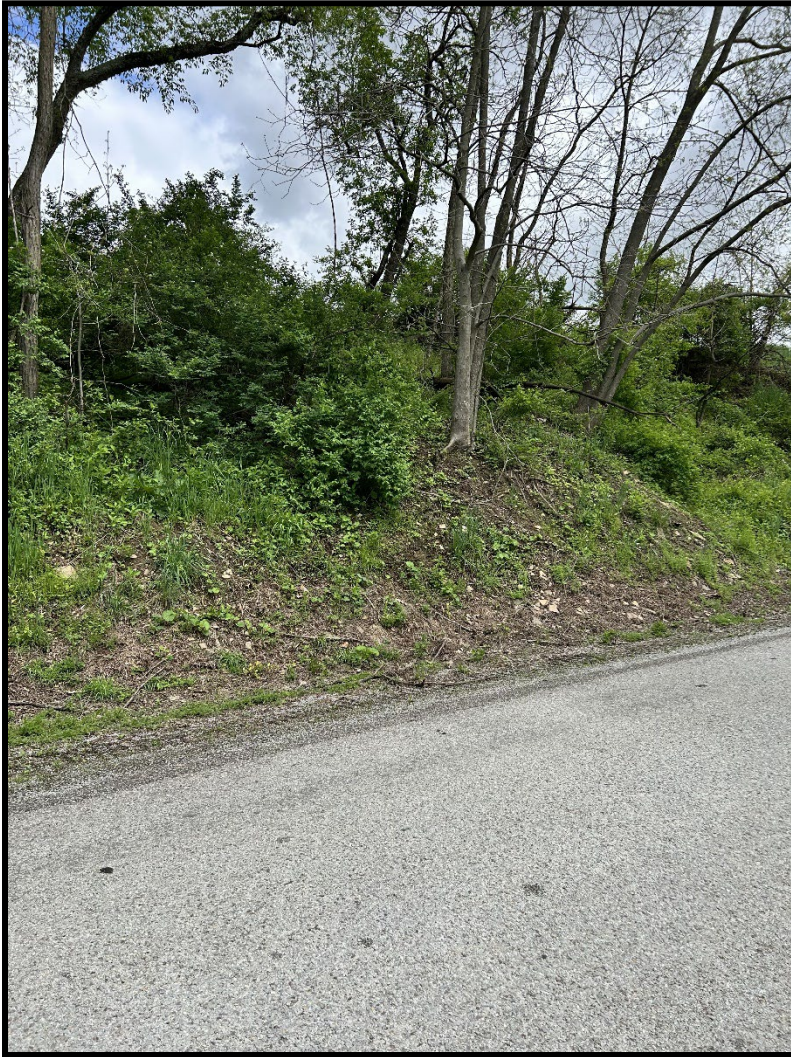
Photograph 18 – Existing Dickey Road crossing cutslope at approximate Station 194+00.
