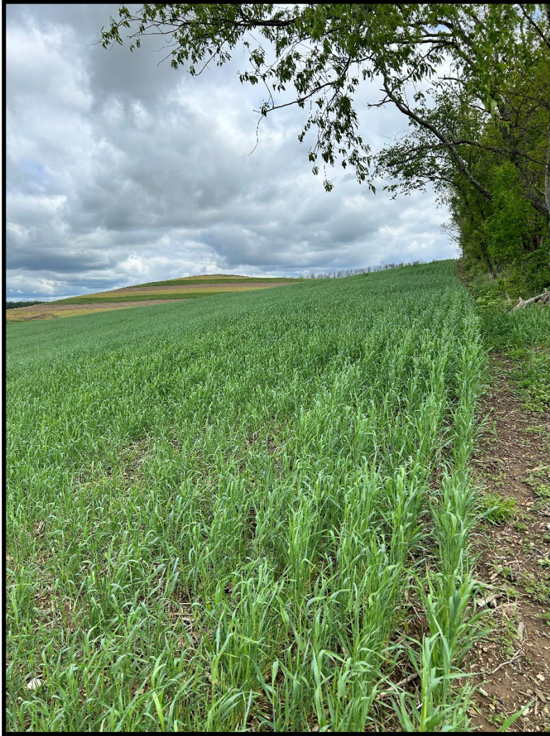
Photograph 13 – View of conditions near approximate Station 153+00.
