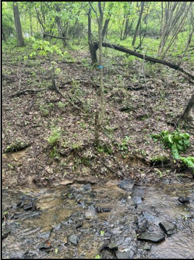
Photograph 2 – View of stream crossing at approximate Station 26+50.
