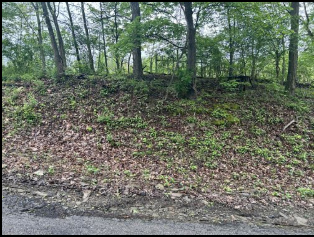
Photograph 6 – Existing slope at Falling Road crossing at approximate Station 55+50.
