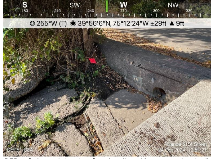
DEP51-S8A sample location. Sample collected from accumulated soil in cracks.
