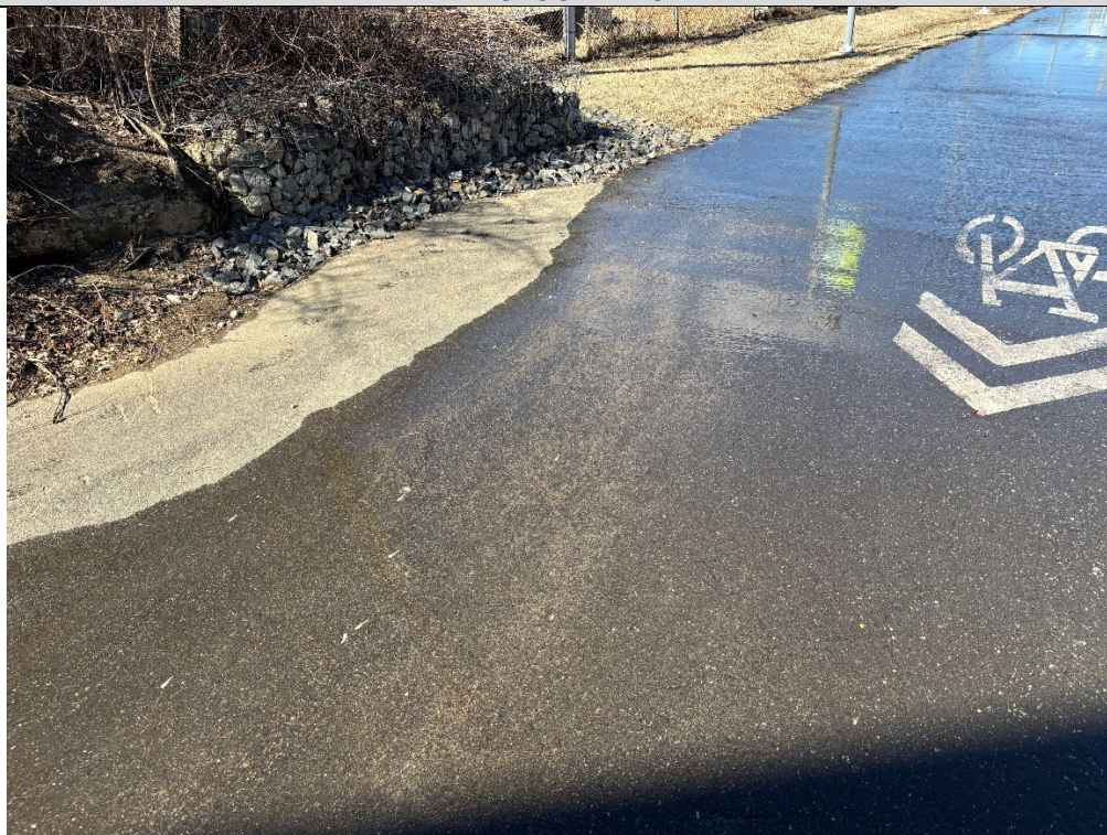
Sediment staining along Bartram's Garden trail. Philadelphia Fire Department was conducting a flushing and/or training activity at a hydrant along 51 st St., causing the wet pavement.
