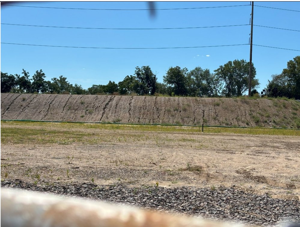
Large fill dirt stockpile with erosion rills and gullies.
