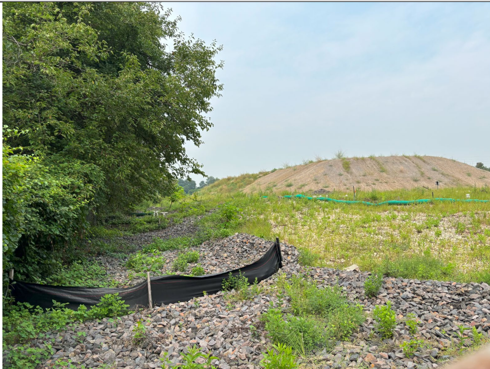
Rock-covered swale, and downslope and back portion (adjacent to railroad tracks) of large fill dirt stockpile.
