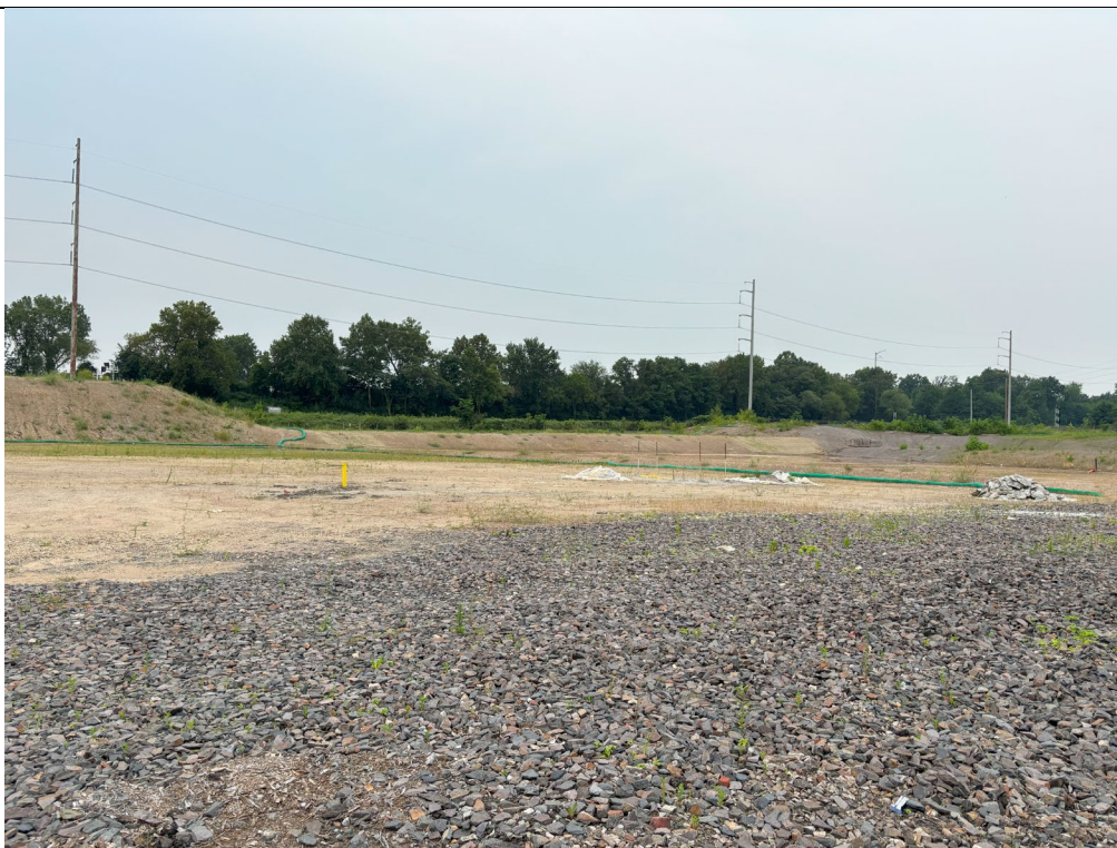
Midslope portion of site showing little stabilization.
