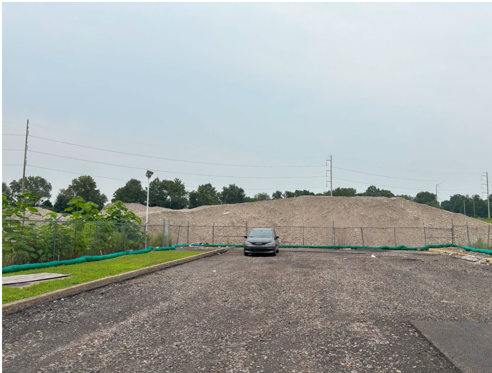
Stone stockpile and filter sock along midslope portion of site, as viewed from 51 st St.
