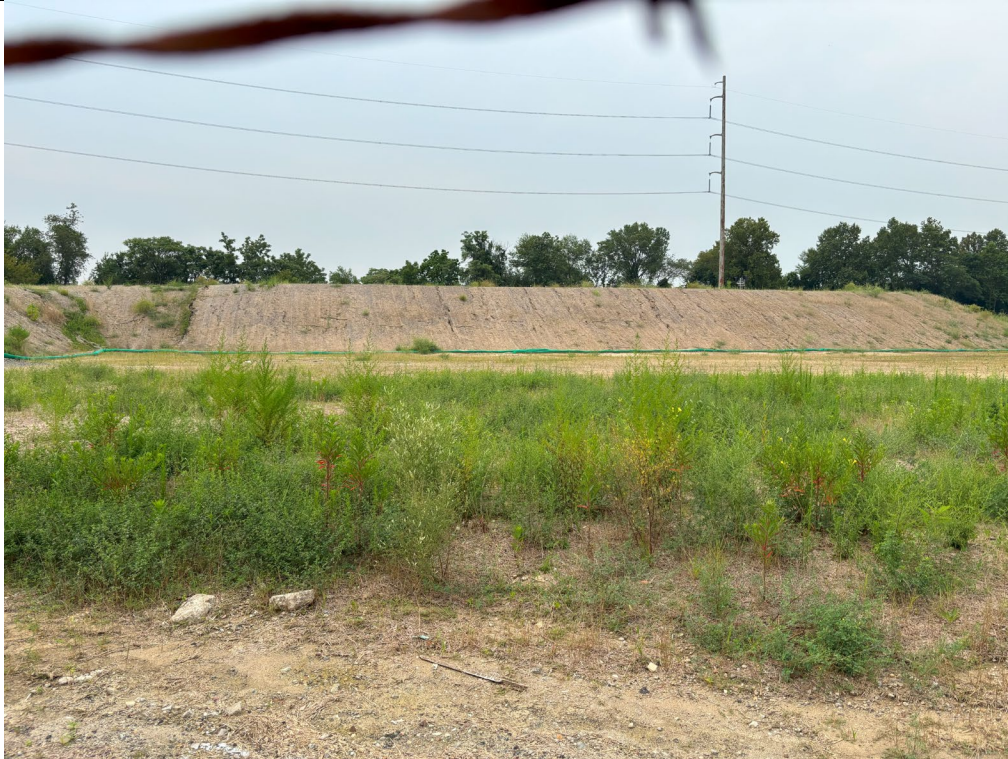
Some stabilized area in foreground; large fill dirt stockpile in distance with some erosion rills and gullies.
