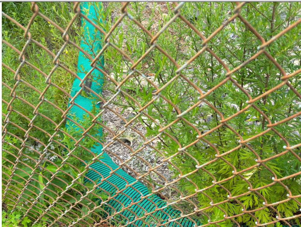
Filter sock at downslope corner of site near 51 st & Botanic Sts.
