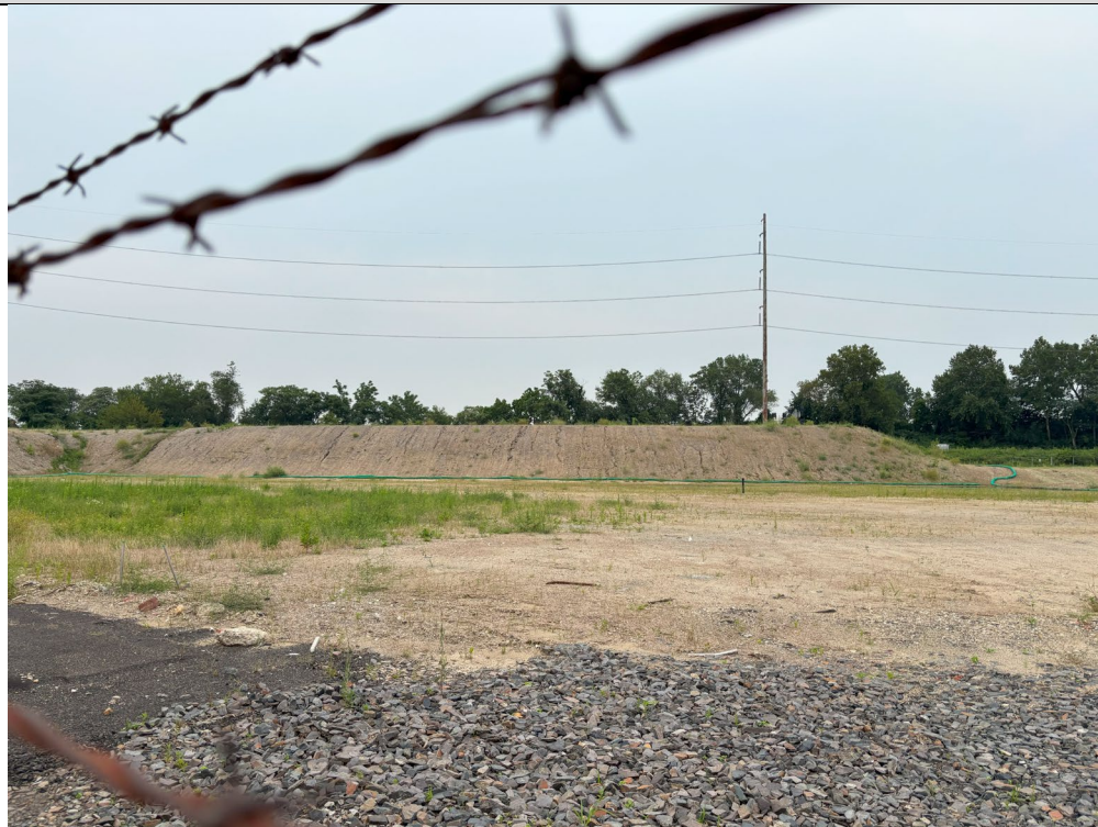
Midslope portion of site with large fill dirt stockpile in background; some erosion rills and gullies present.
