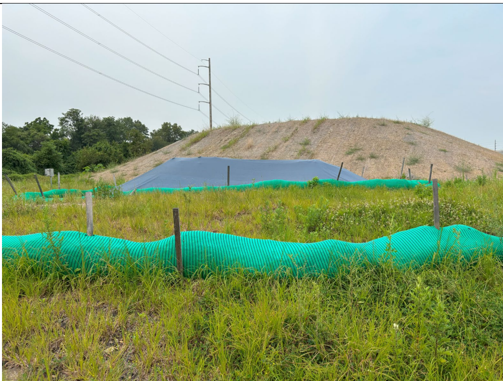
Downslope filter sock with tarped contaminated dirt stockpile and downslope end of large fill dirt stockpile in distance.
