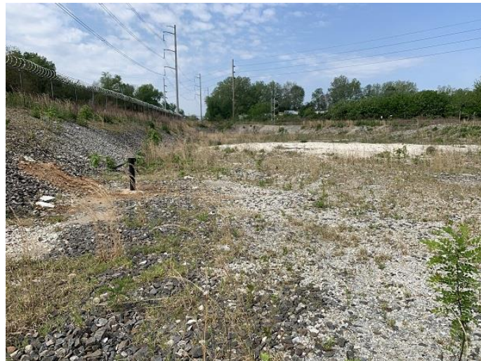
MW-9 and deposited fill in the upgradient tank containment
