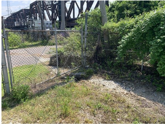
Ditch at the property fence line.
