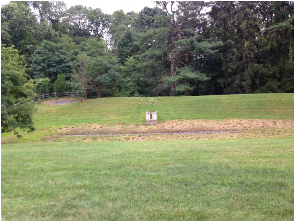
44. View east of emergent wetlands (C20) in a stormwater management basin within the ROW of the pipeline within Parcel PA-DE-0059.0000 (September 9, 2014).
