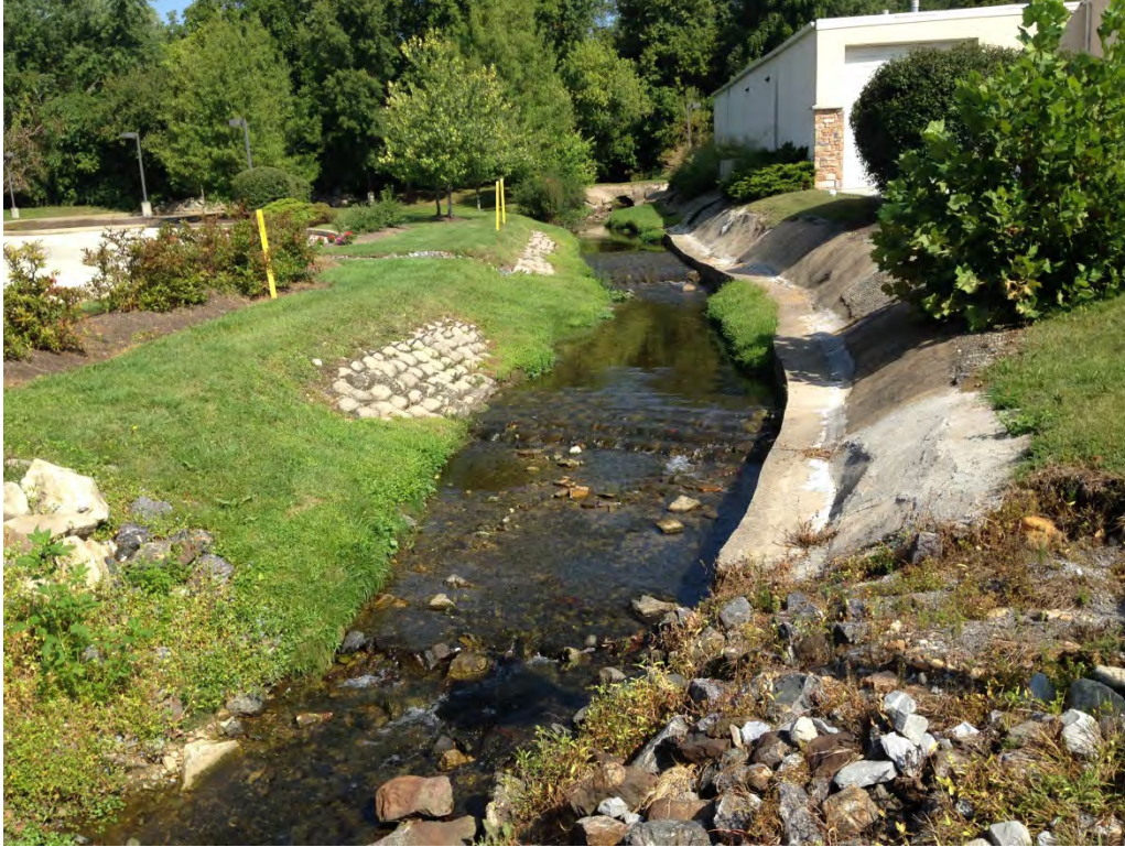
25. View north of a historically disturbed small stream channel (S-C59) within the ROW of the pipeline within Parcel PA-CH-0212.0000-WX (September 2, 2014).
