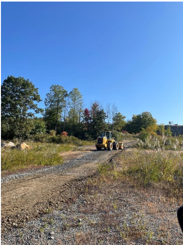
Front-end loader leveling road - 10/11/22, 9:56 AM
