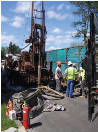
Drill rig over recovery well RW-2 5-19-25 @ 15:25
