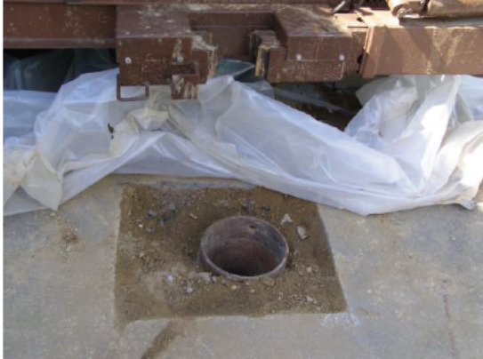
Recovery well RW-2 with auger to keep from caving in 5-19-25 @ 16:14
