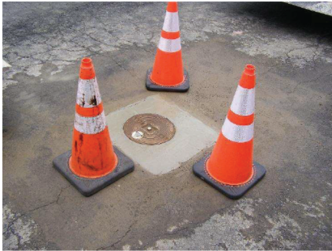
Photo 5: Concrete pad installation at RW-2
