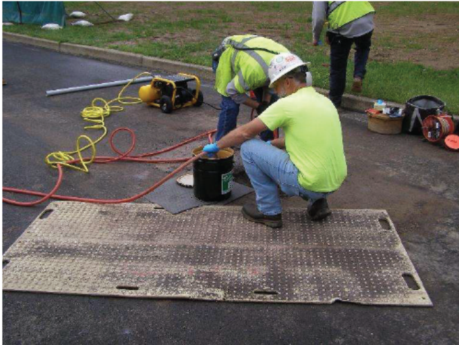
Photo 1: Pneumatic pump used to collect LNAPL in RW-3
