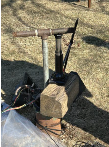
128 Walker Road potable well 2-24-25 @ 10:07
