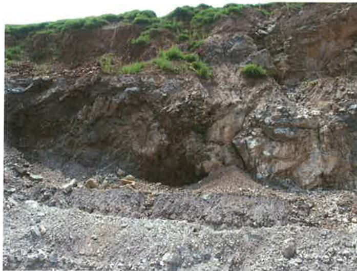
Fault zone (south wall, dry)
