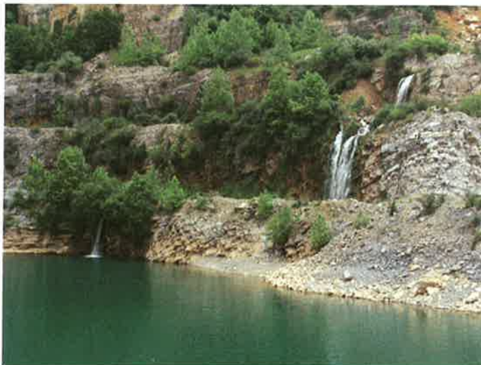
Culvert (northwest corner of sump); Primrose Creek outflow on west wall
