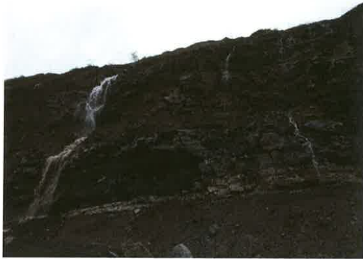
Fault zone (looking up from base of highwall)
