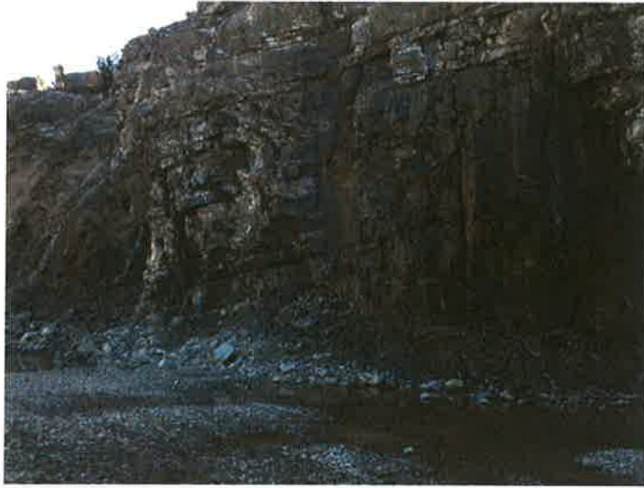
Southeast Wall (behind sump transducer, wall very wet)
