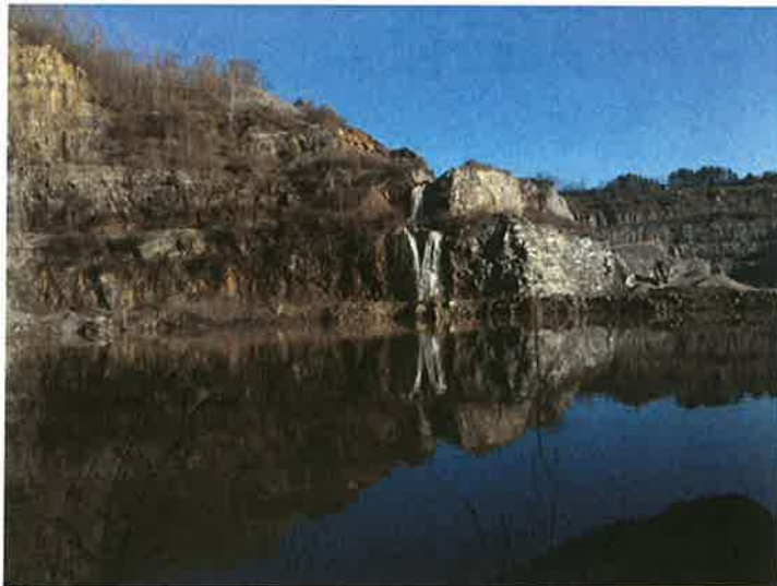
Looking North across sump to Primrose Creek outflow on west wall
