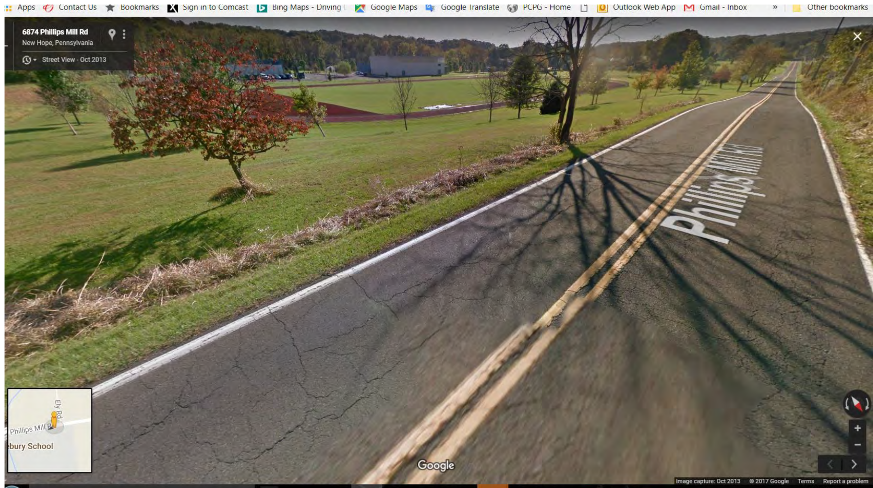
Figure 4 2013 Google Street View. Looking SW. Feature “A” by tree on Right, Feature “C” on left by tree. Similar to as observed in 2017. Line in ground appears to be runoff from Phillips Mill Road
