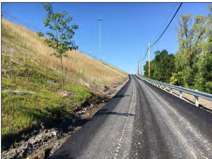
Figure 2. Paved access road and stabilized landfill slope.
