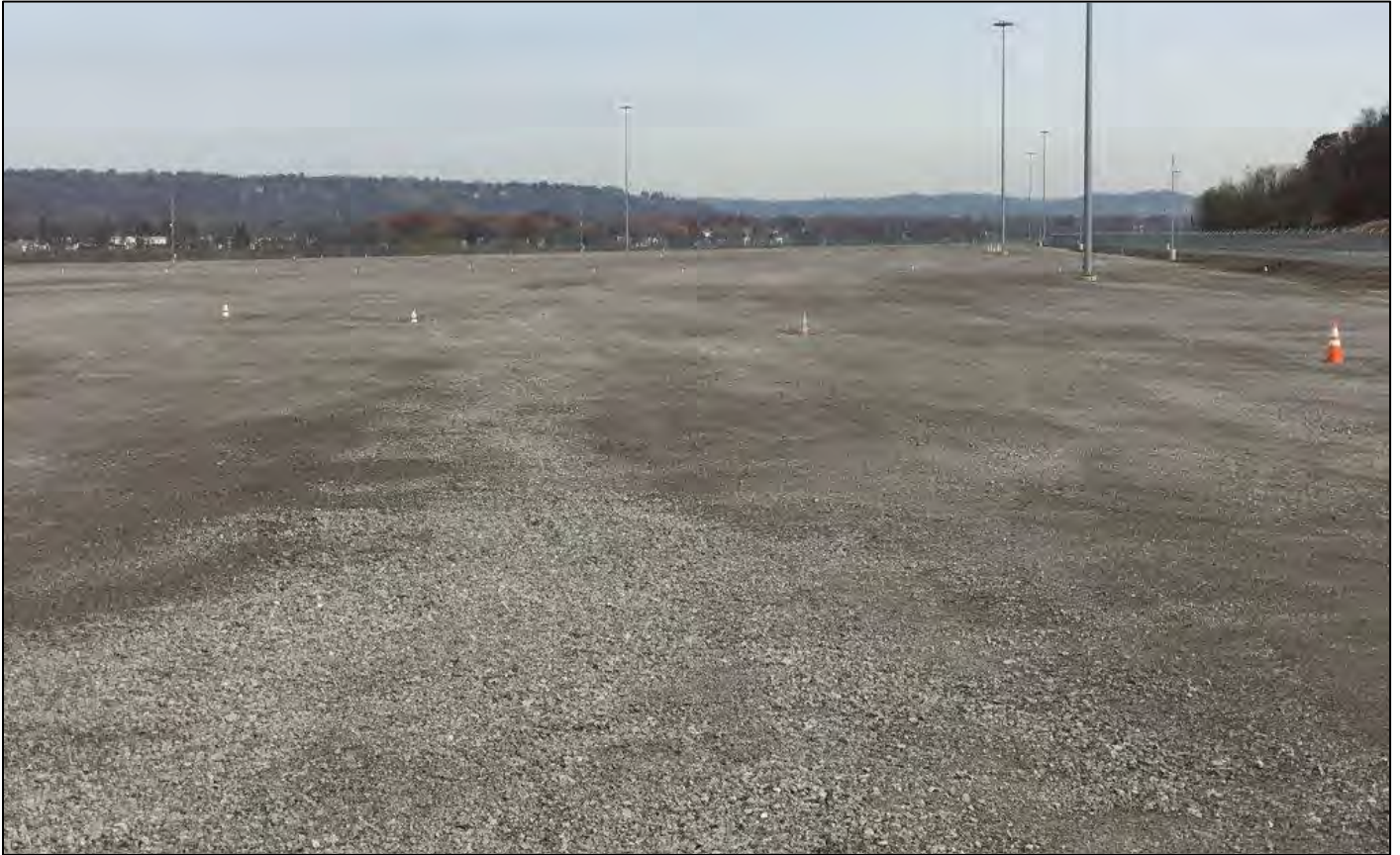
Figure 6. Fly Ash Landfill area after re-grading and placement of geotextile and structural stone. (2018)
