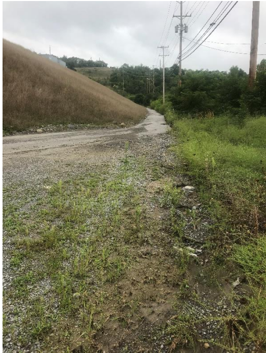
Improved vegetation vicinity Outfall 021; view uphill from outfall
