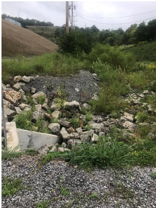
Rip rap and vegetation Outfall 021
