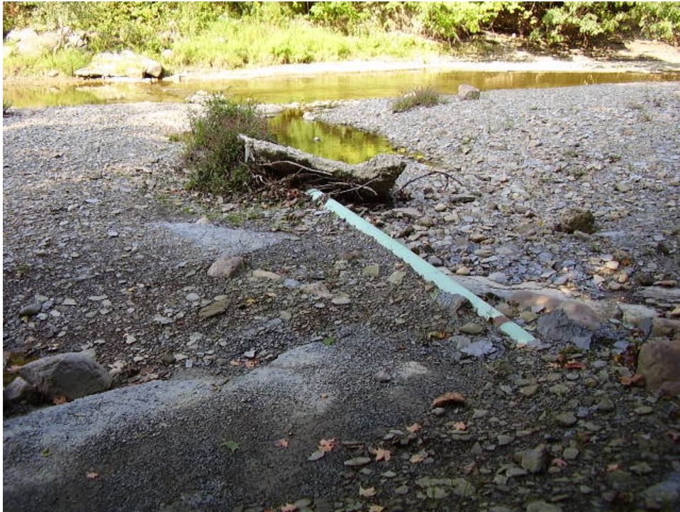
Photo 40 – Exposed Pipe, Upstream Millfair Road Bridge
