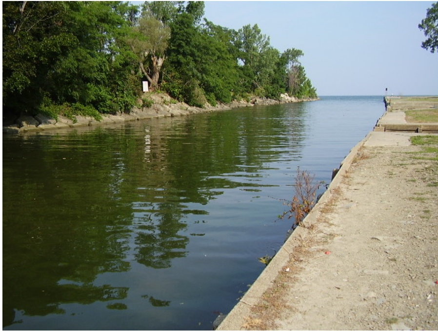
Photo 1 – Channel Alteration / Inadequate Buffer at the mouth of Walnut Creek
