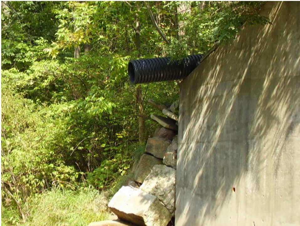
Photo 35 – Channel Alteration / Pipe Outfall, Downstream Millfair Road Bridge
