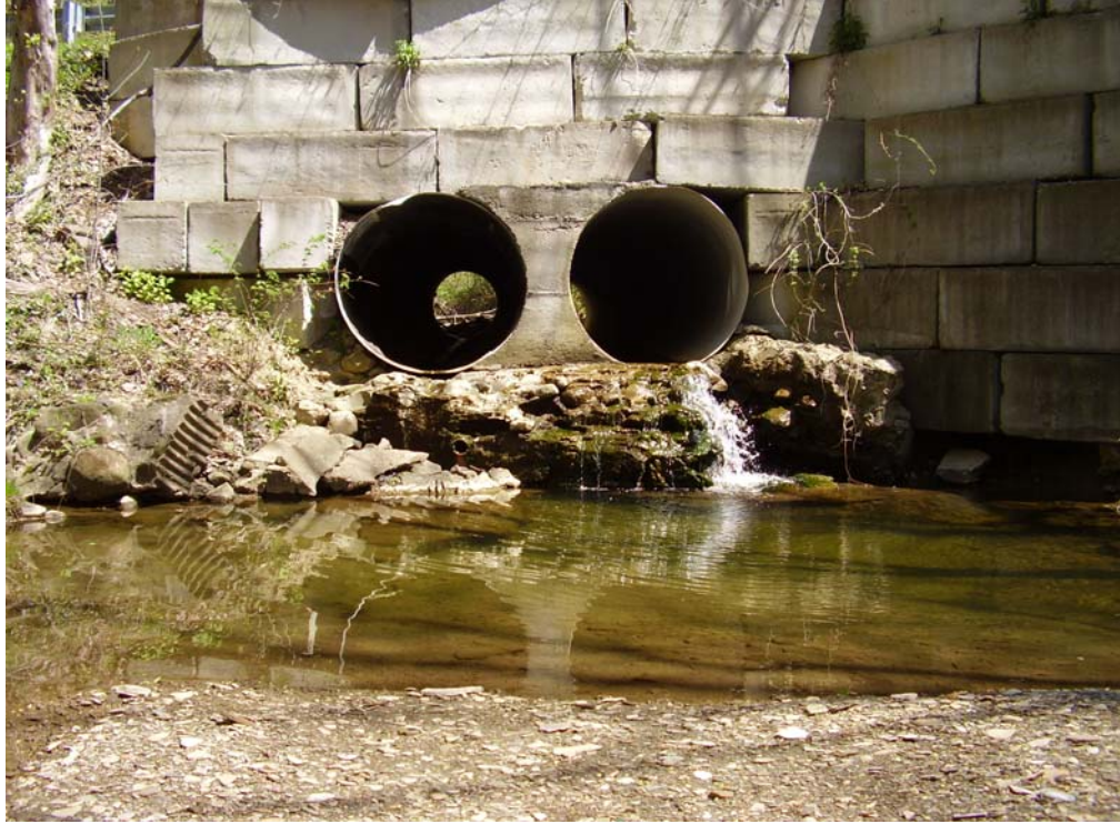
Photo 64 - Obstructions to Fish Passage (15UNT).
