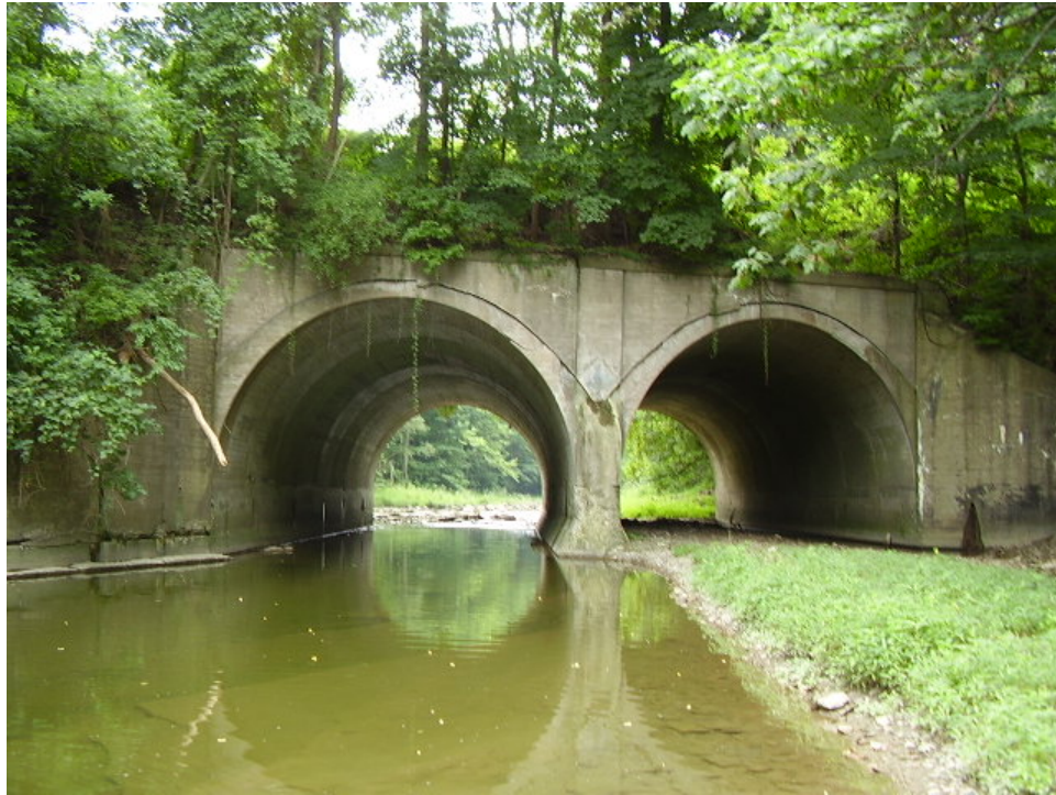
Photo 19 – Channel Alteration / Sedimentation, Downstream U.S. Highway 5 Bridge
