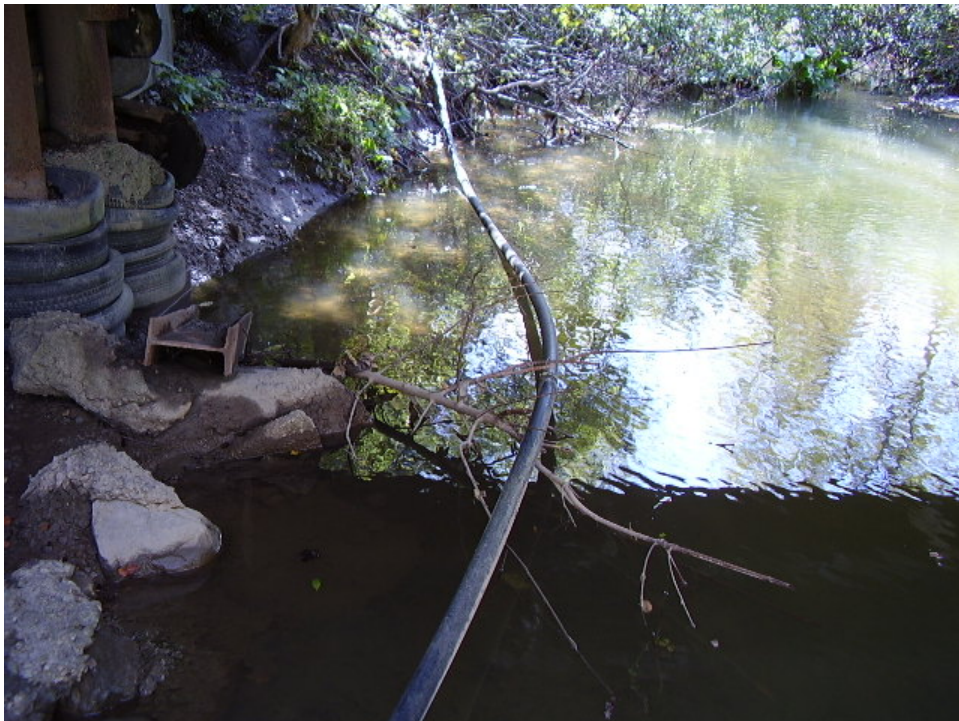
Photo 78 – Exposed Pipe / Channel Alteration
