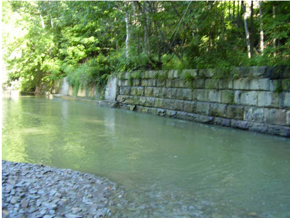
Photo 24 – Channel Alteration / Sedimentation, Downstream CSXT RR Bridge
