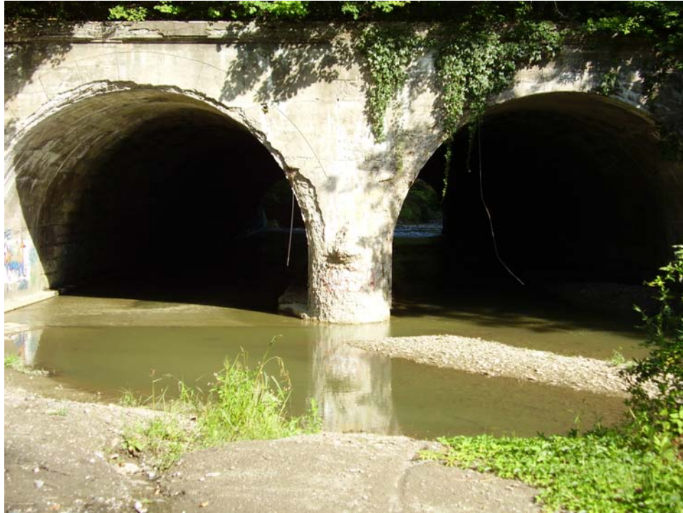
Photo 20 – Channel Alteration / Sedimentation, Downstream CSXT RR Bridge
