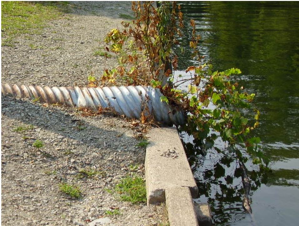
Photo 2 – Exposed Pipe, PFBC Manchester Facility
