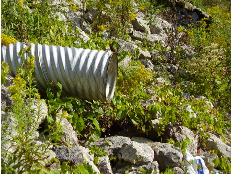
Photo 62 – Pipe Outfall, Interstate 79 Bridge Crossing
