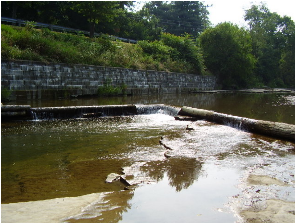
Photo 6 – Channel Alteration for habitat improvement/ potential fish barrier, PFBC Manchester Facility
