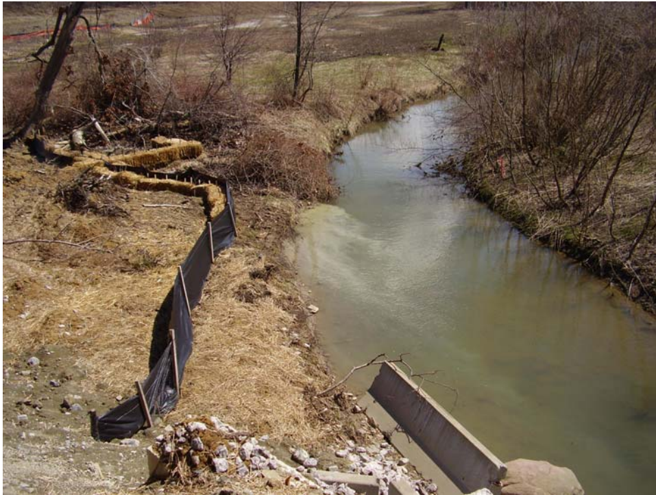
Photo 79 – Channel Alteration / Inadequate Buffer
