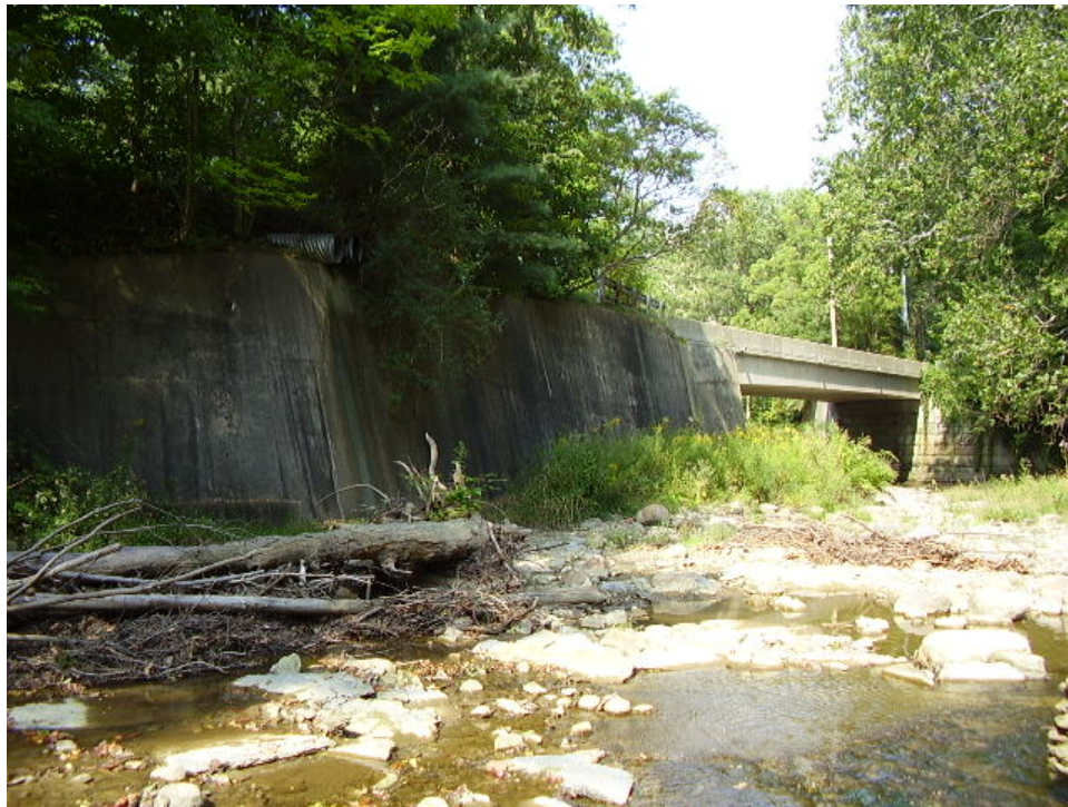
Photo 36 – Channel Alteration, Upstream Millfair Road Bridge
