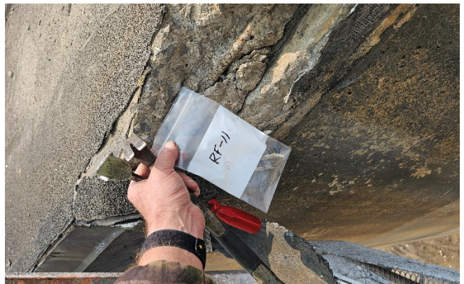
Photo 22: SAMPLE RF-11 UNIT #1 TOP ASH SILO FLASHING
