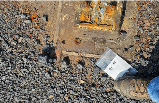
Photo 3: SAMPLE RF-01 CAULKING SILO 1
