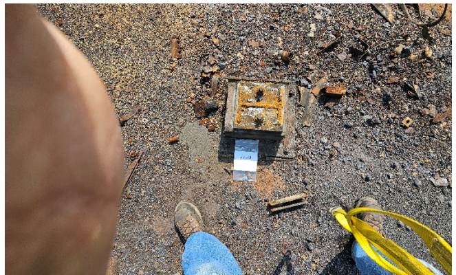
Photo 4: SAMPLE RF-02 CAULKING SILO 1
