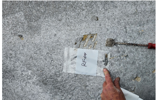
Photo 14: SAMPLE RF-04 LIME SILOS 1&2 A&B ROOFING
