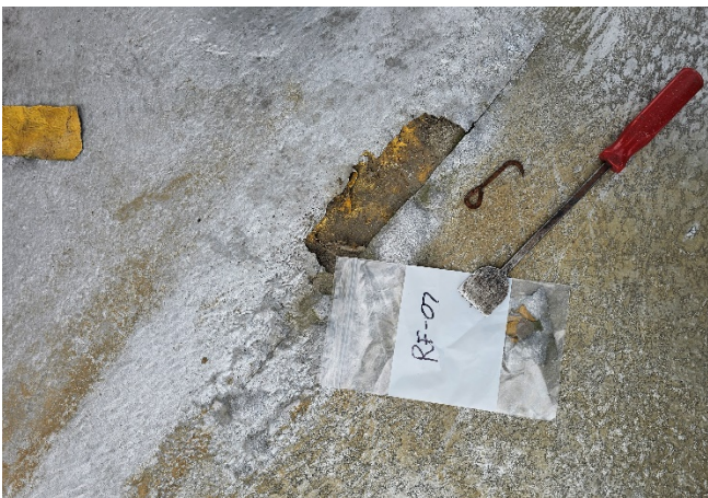
Photo 17: SAMPLE RF-07 BYPRODUCT SILOS 1&2 ROOFING
