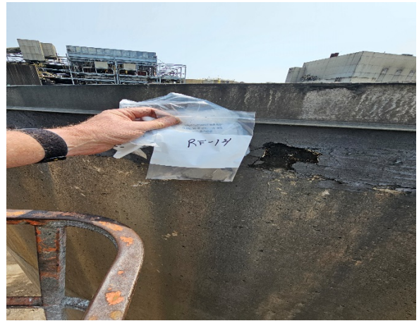
Photo 26: SAMPLE RF-14 UNIT #2 TOP ASH SILO FLASHING
