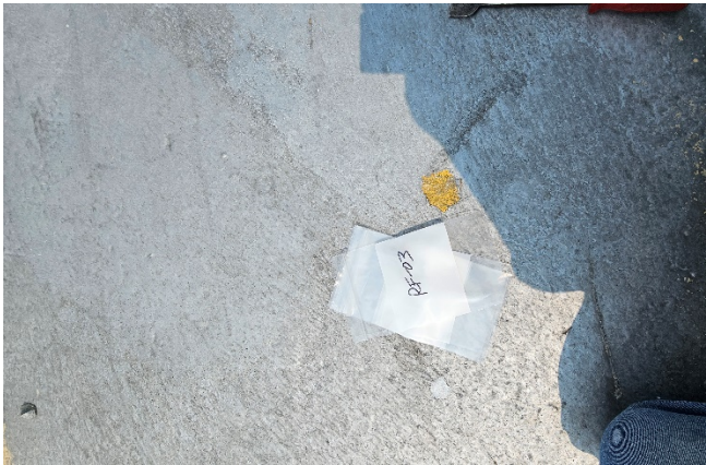
Photo 13: SAMPLE RF-03 LIME SILOS 1&2 A&B ROOFING
