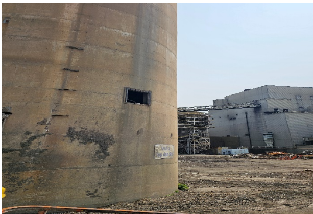
Photo 23: UNIT #2 TOP ASH SILO
