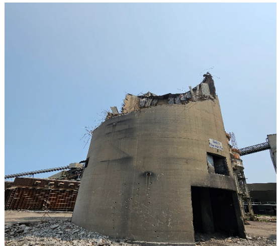
Photo 28: UNIT #3 TOP ASH SILO
