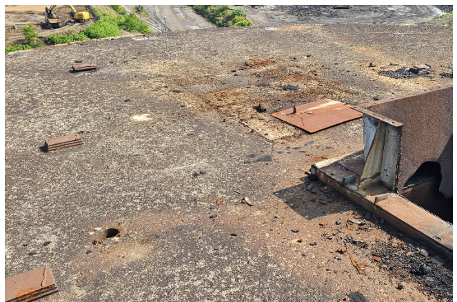
Photo 6: TOP OF SILO 3 NO VISIBLE SUSPECT ACMS
