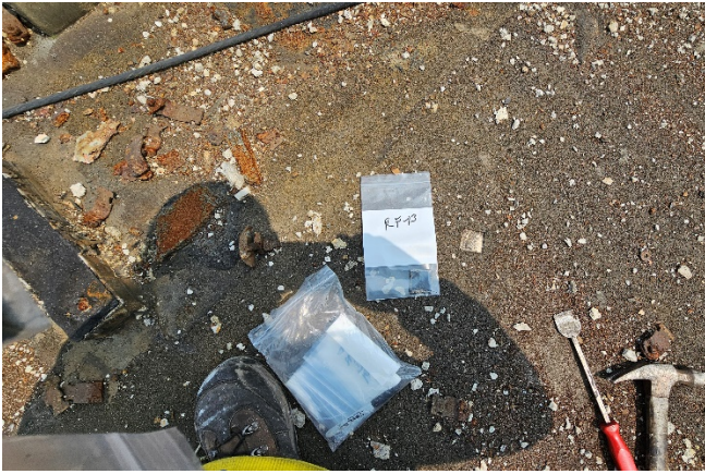
Photo 25: SAMPLE RF-13 UNIT #2 TOP ASH SILO ROOFING
