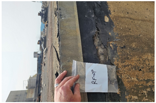
Photo 20: SAMPLE RF-09 UNIT #1 TOP ASH SILO FLASHING
