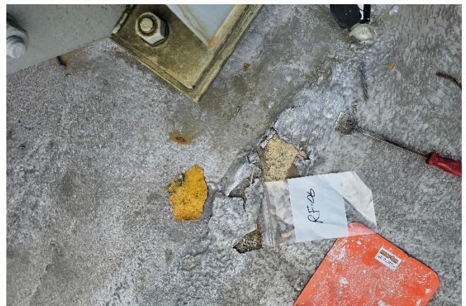
Photo 16: SAMPLE RF-06 BYPRODUCT SILOS 1&2 ROOFING
