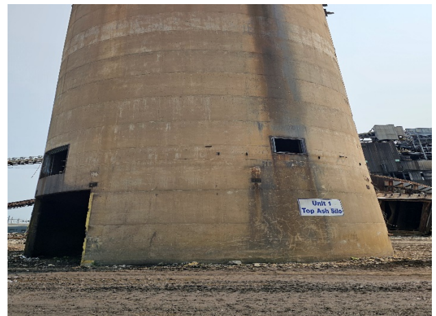
Photo 18: UNIT #1 TOP ASH SILO
