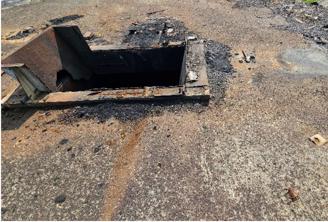
Photo 7: TOP OF SILO 3 NO VISIBLE SUSPECT ACMS
