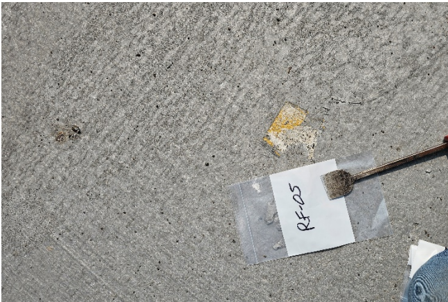
Photo 15: SAMPLE RF-05 LIME SILOS 1&2 A&B ROOFING
