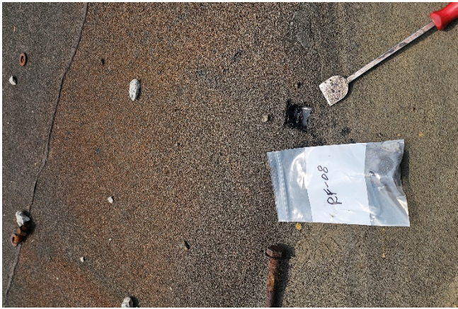
Photo 19: SAMPLE RF-08 UNIT #1 TOP ASH SILO ROOFING
