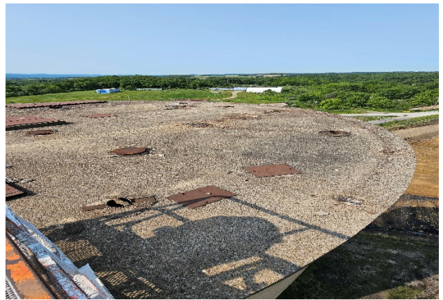
Photo 10: TOP OF SILO 5 NO VISIBLE SUSPECT ACMS
