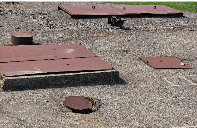
Photo 11: TOP OF SILO 5 NO VISIBLE SUSPECT ACMS
