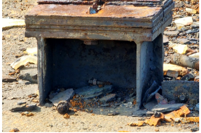
Photo 8: TOP OF SILO 4 NO VISIBLE SUSPECT ACMS
