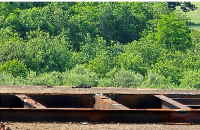
Photo 9: TOP OF SILO 4 NO VISIBLE SUSPECT ACMS
