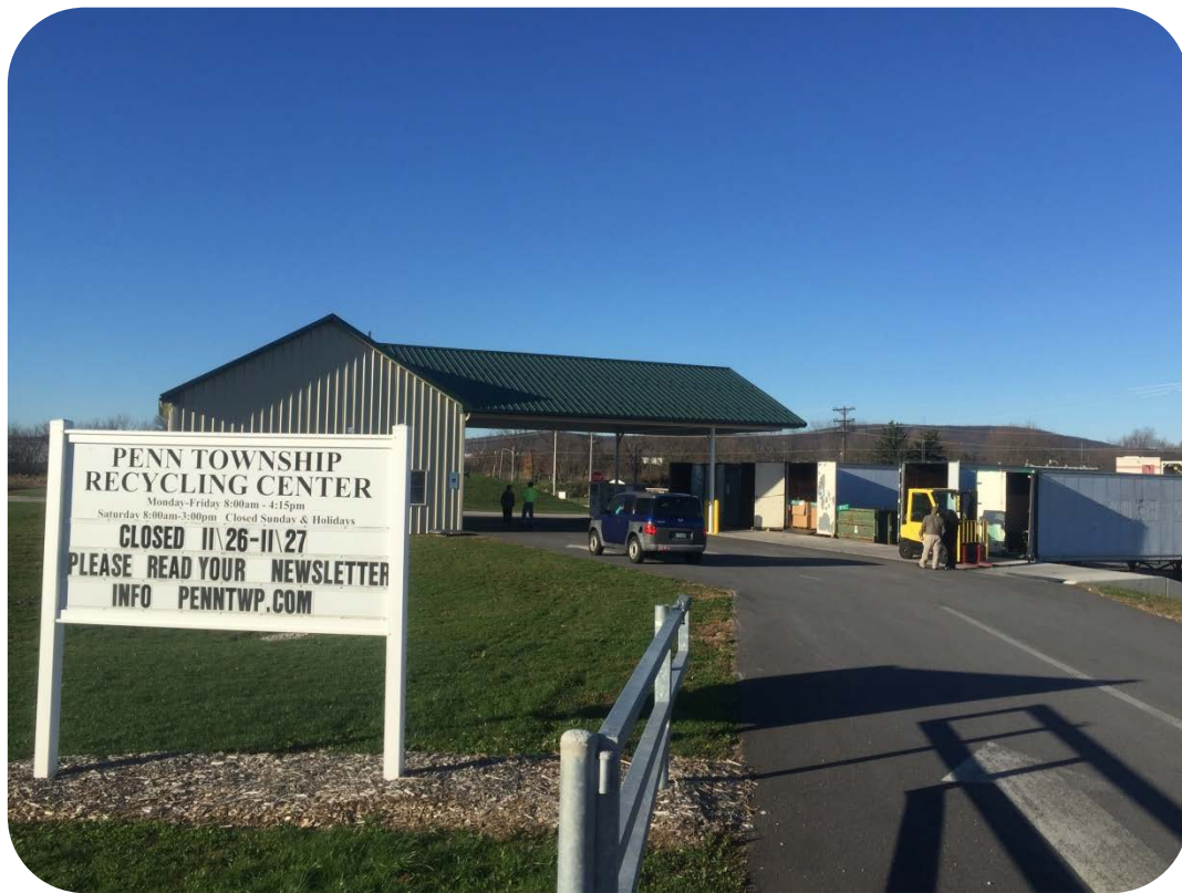
Penn Township Recycling Center Photo Source: Gannett Fleming, Inc.
