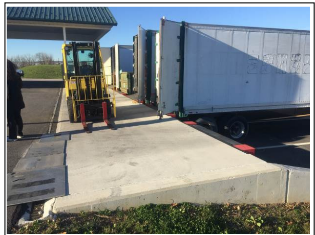
Photo 10: 11-20-15. Penn Township Drop-off Facility Loading Dock (8 bays)
