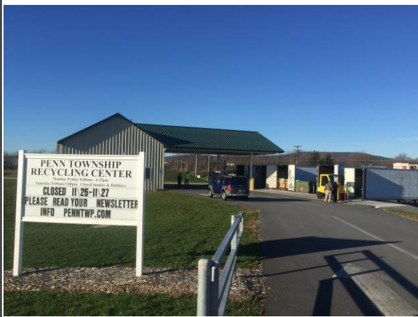
Photo 7: 11-20-15. Penn Township Drop-off Facility Facility Entrance (3 lanes wide)
