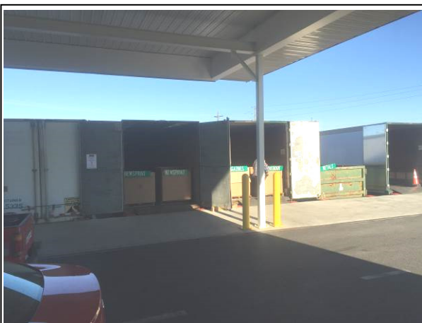
Photo 11: 11-20-15. Penn Township Drop-off Facility Drive through – Vehicle Unload Area
