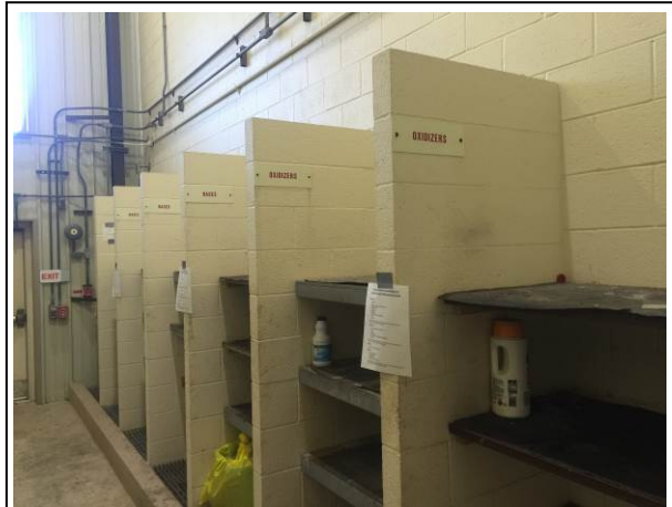
Photo 4: 11-20-15. LCSWMA Chemical Storage Bays
