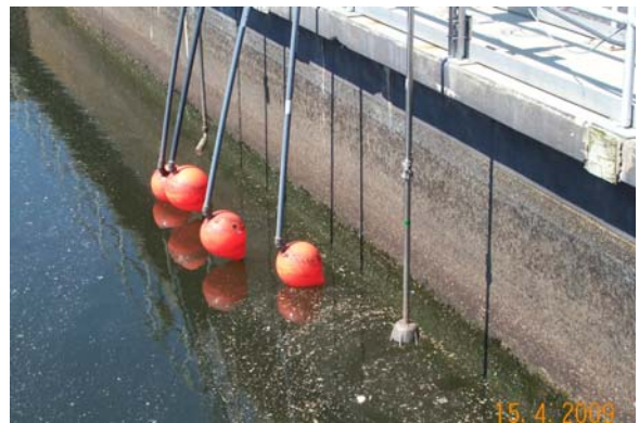
Figure F.6: Probes during decant cycle, two are above water.
