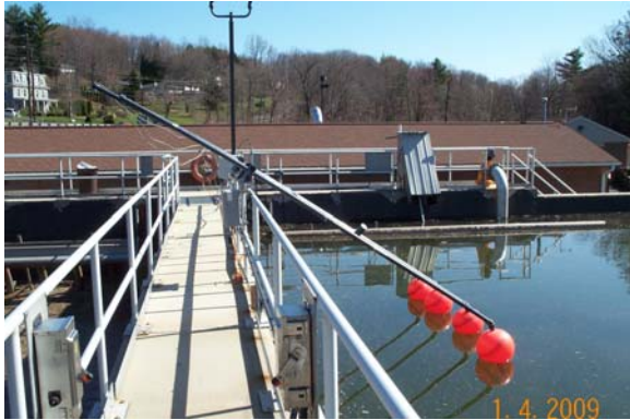
Figure F.7: Probe floats at high-level/start of decant cycle.
